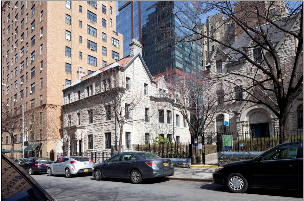
St. Michael's Rectory 227 West 99 th Street, Block 1871 Lot 24 Photographs: Marianne S. Percival, 2016
