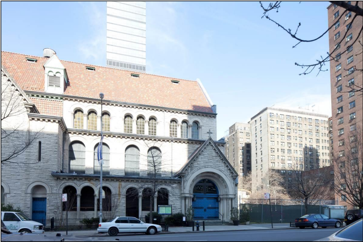
St. Michael's Church, east elevation Photographs: Marianne S. Percival, 2016
