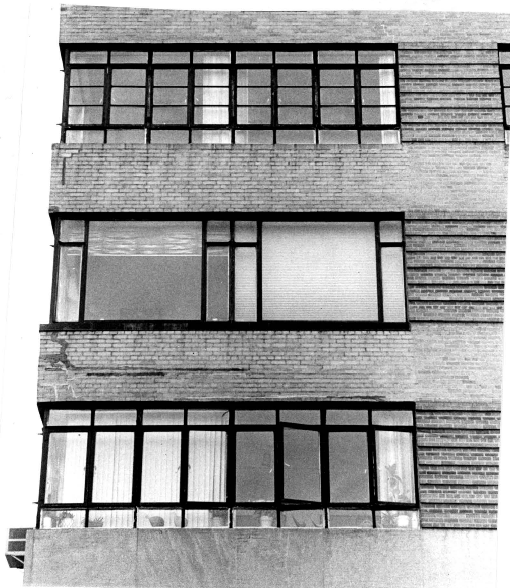
Majestic Apartments: Views of the corners of the building, with setbacks, brick paneling, and metal railings. The wrap-around windows with triple panes show the original configuration.
