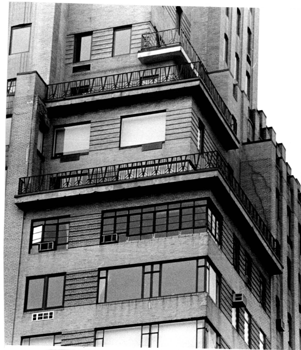
Majestic Apartments: Views of the corners of the building, with setbacks, brick paneling, and metal railings. The wrap-around windows with triple panes show the original configuration.
