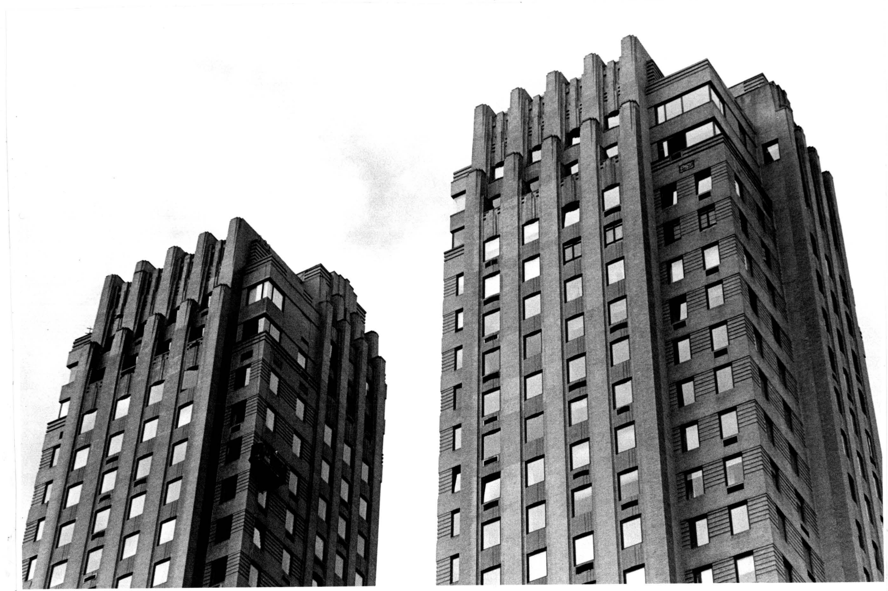
Majestic Apartments: View of the twin towers, with window alterations.
