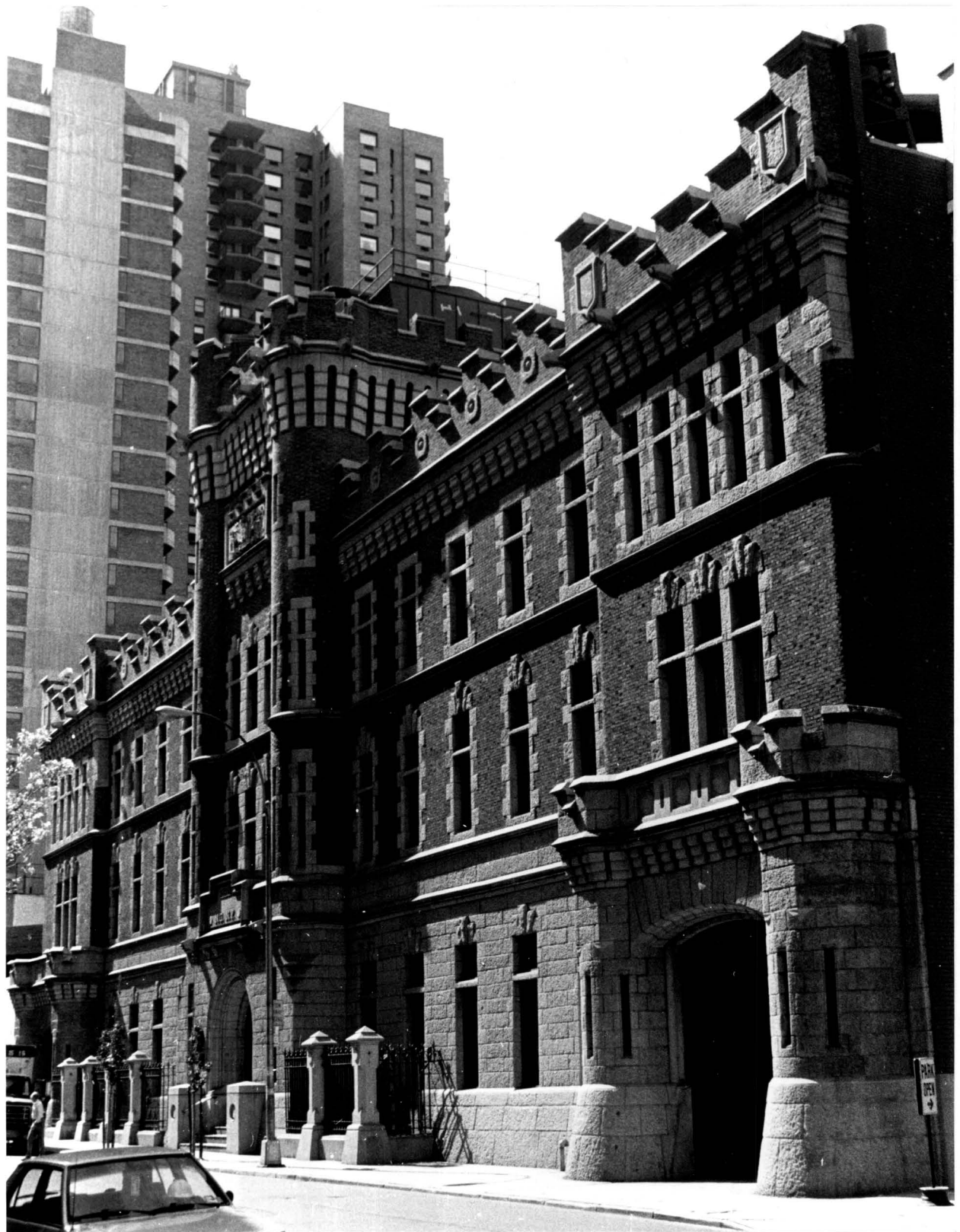
First Battery Armory, 1900-1903 56 West 66th Street, Manhattan
