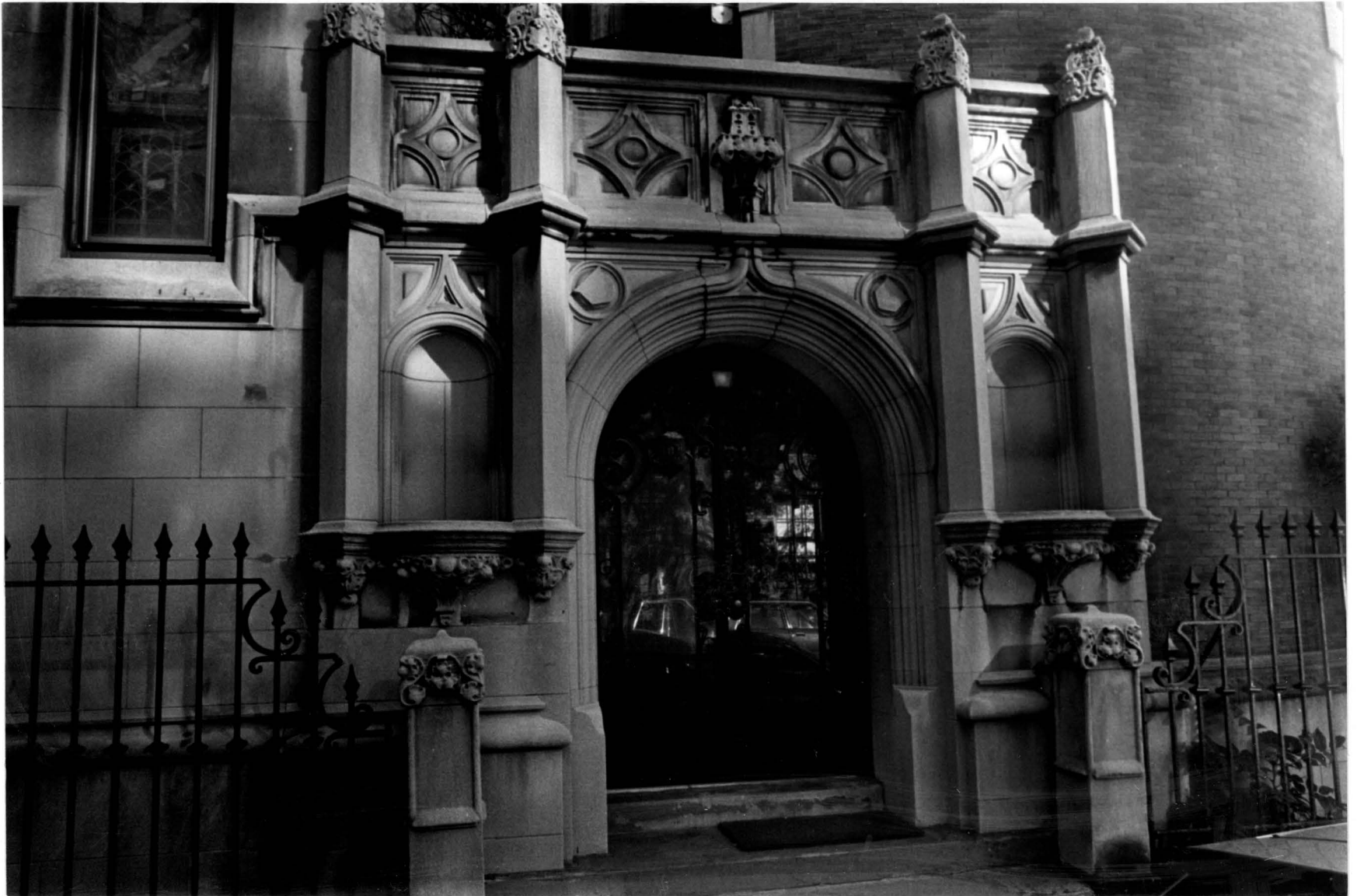
107-109 Riverside Drive Entrance
