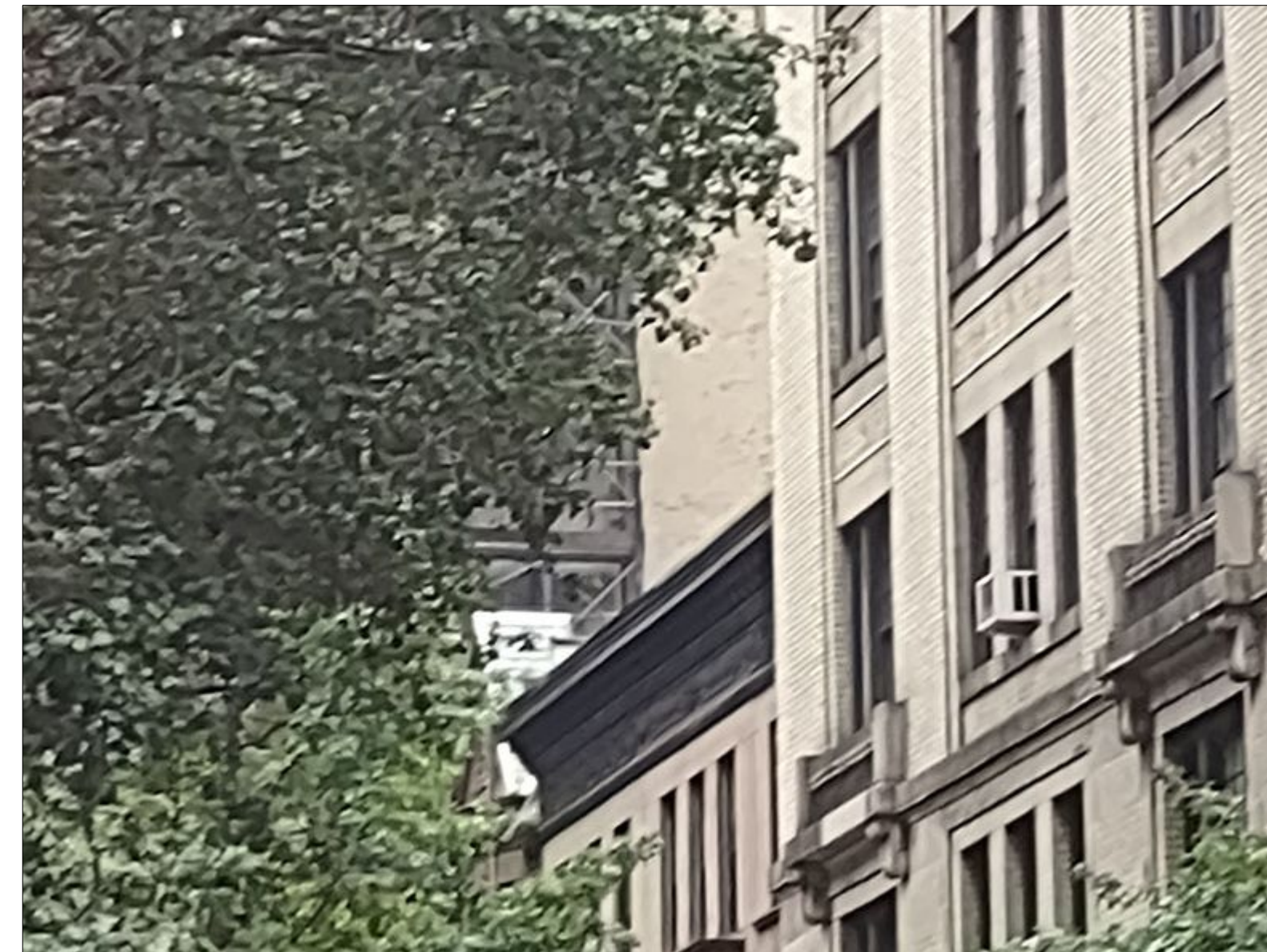
LOOKING SOUTH EAST- CLOSE UP
