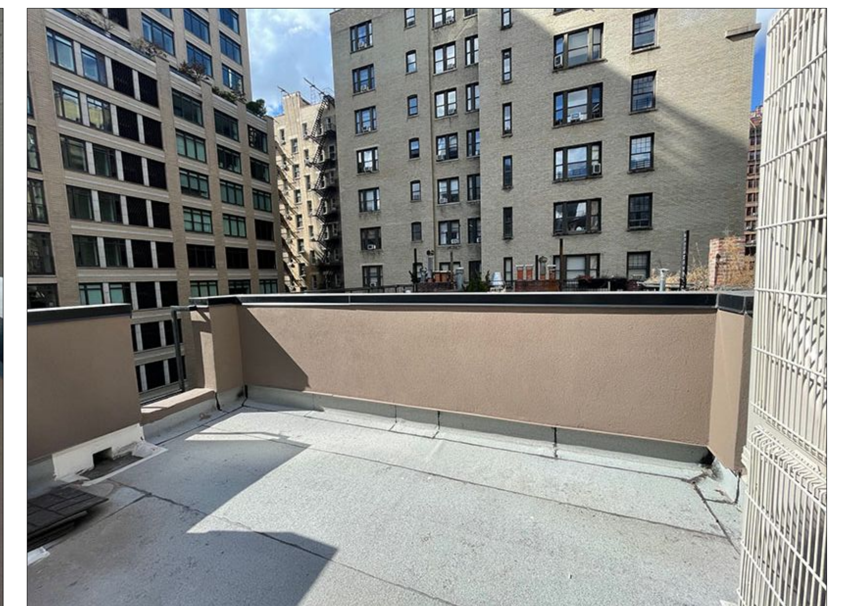
ADDITION ROOF- LOOKING EAST
