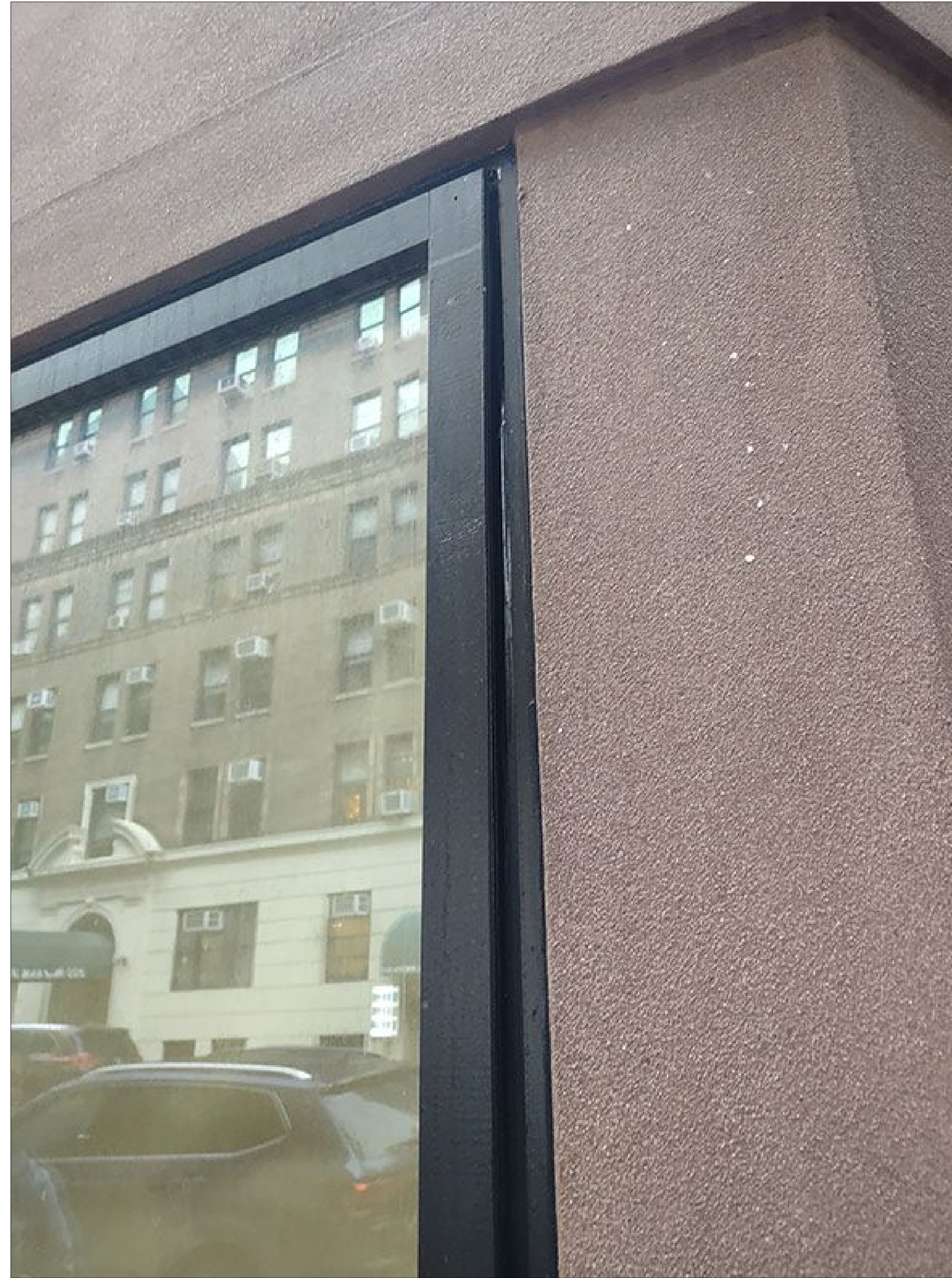
N.E. BASEMENT BAY CORNER
