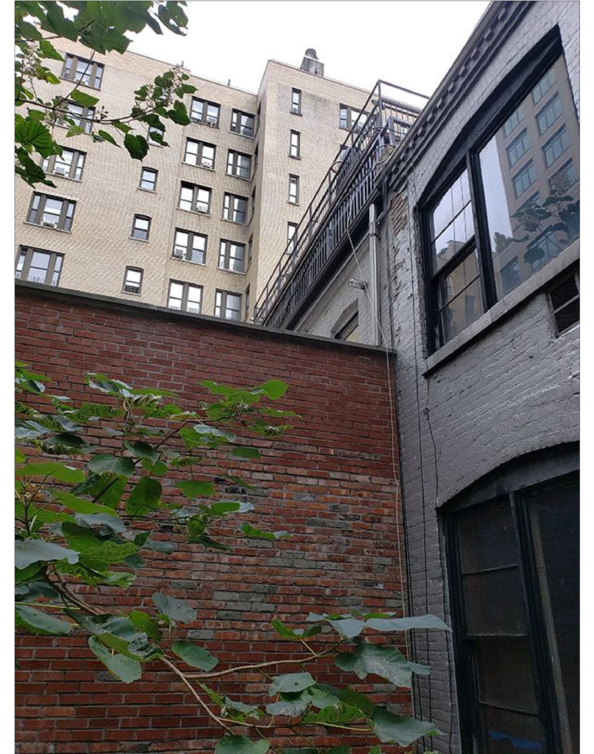
NEIGHBORING SOUTH FACADE LOOKING WEST
