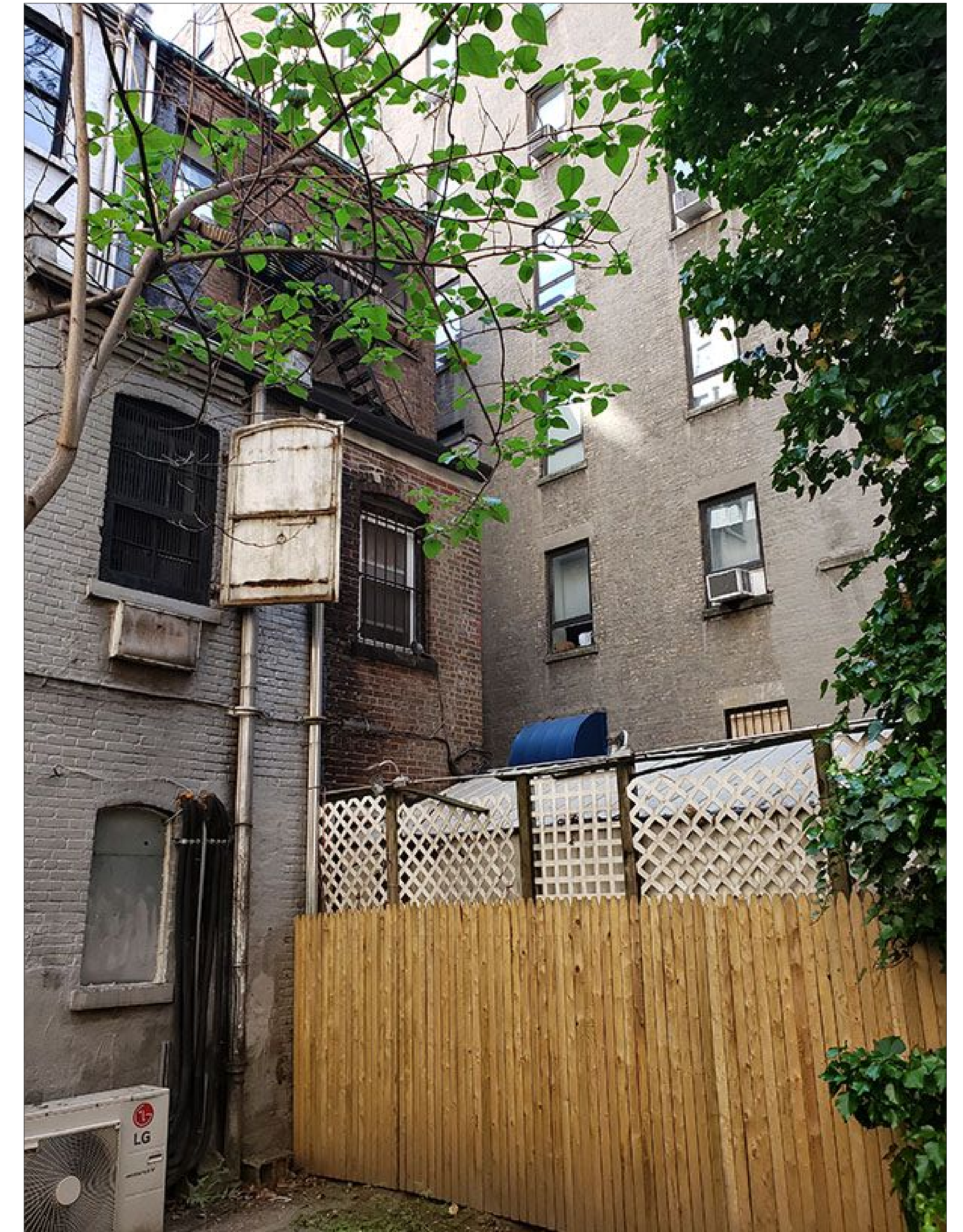
SOUTH FACADES IN CONTEXT
