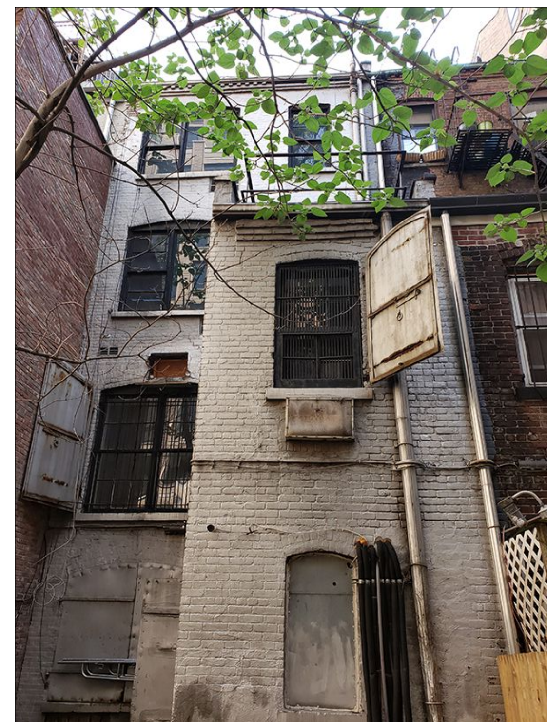
EXISTING SOUTH FACADE
