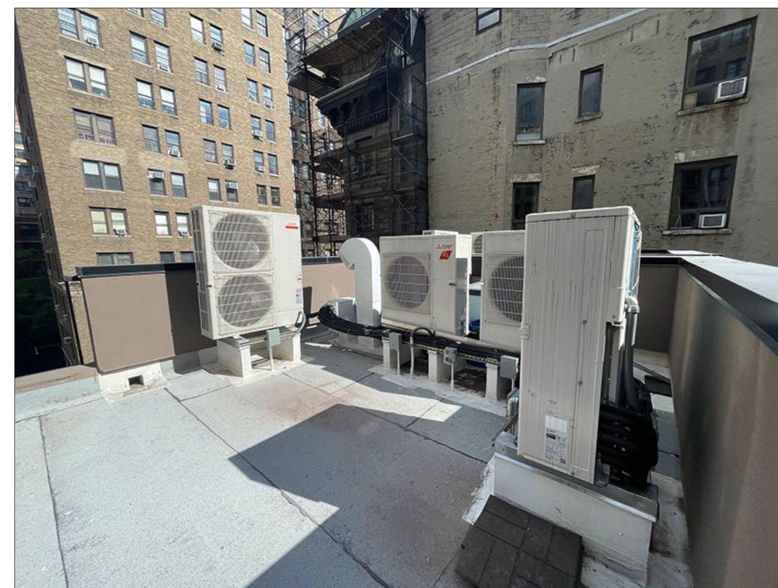
ADDITION ROOF- LOOKING NORTH WEST
