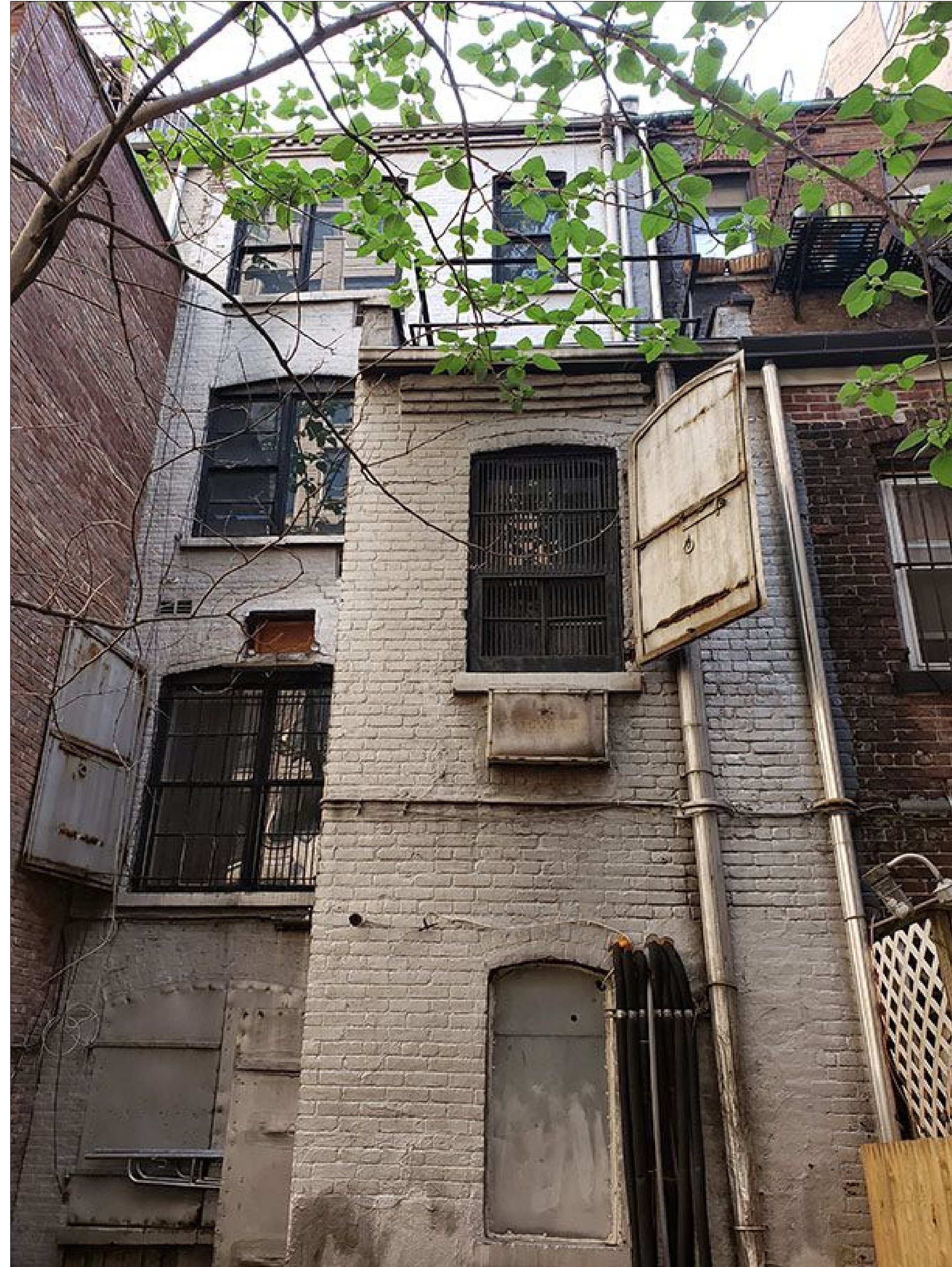
SOUTH FACADE PRIOR TO CONSTRUCTION
