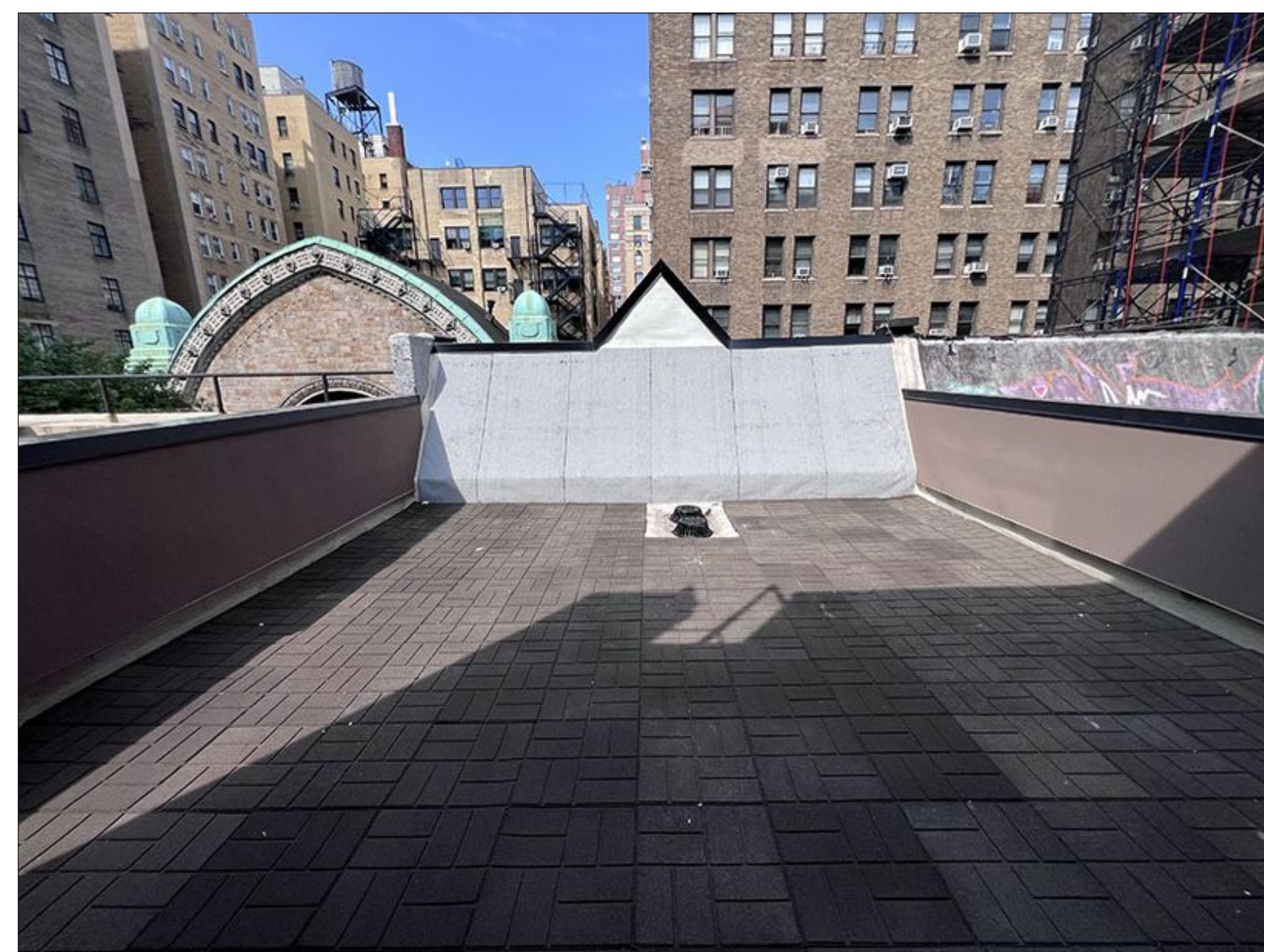
PENTHOUSE ROOF- LOOKING NORTH
