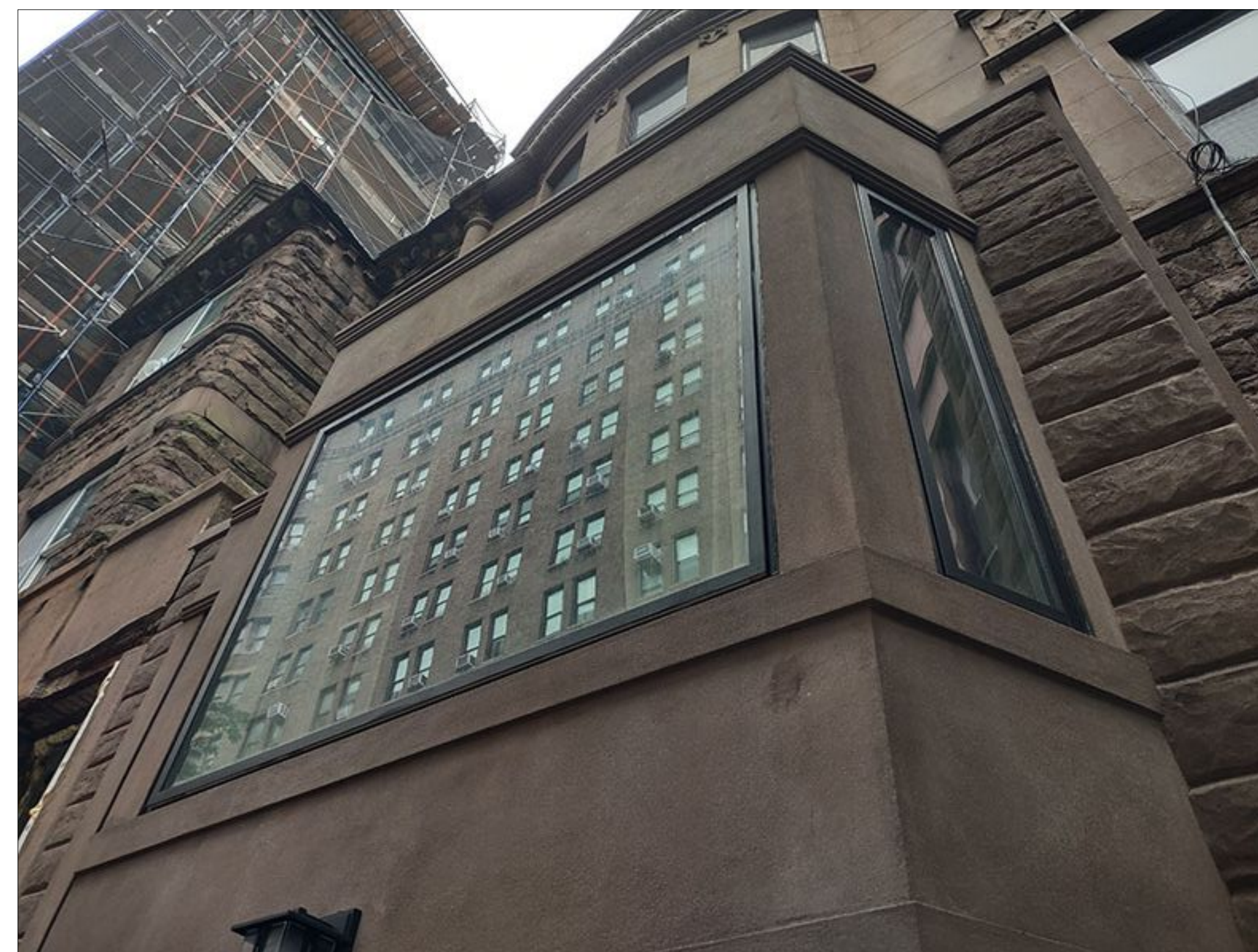
N.E 1ST FLOOR BAY WINDOWS
