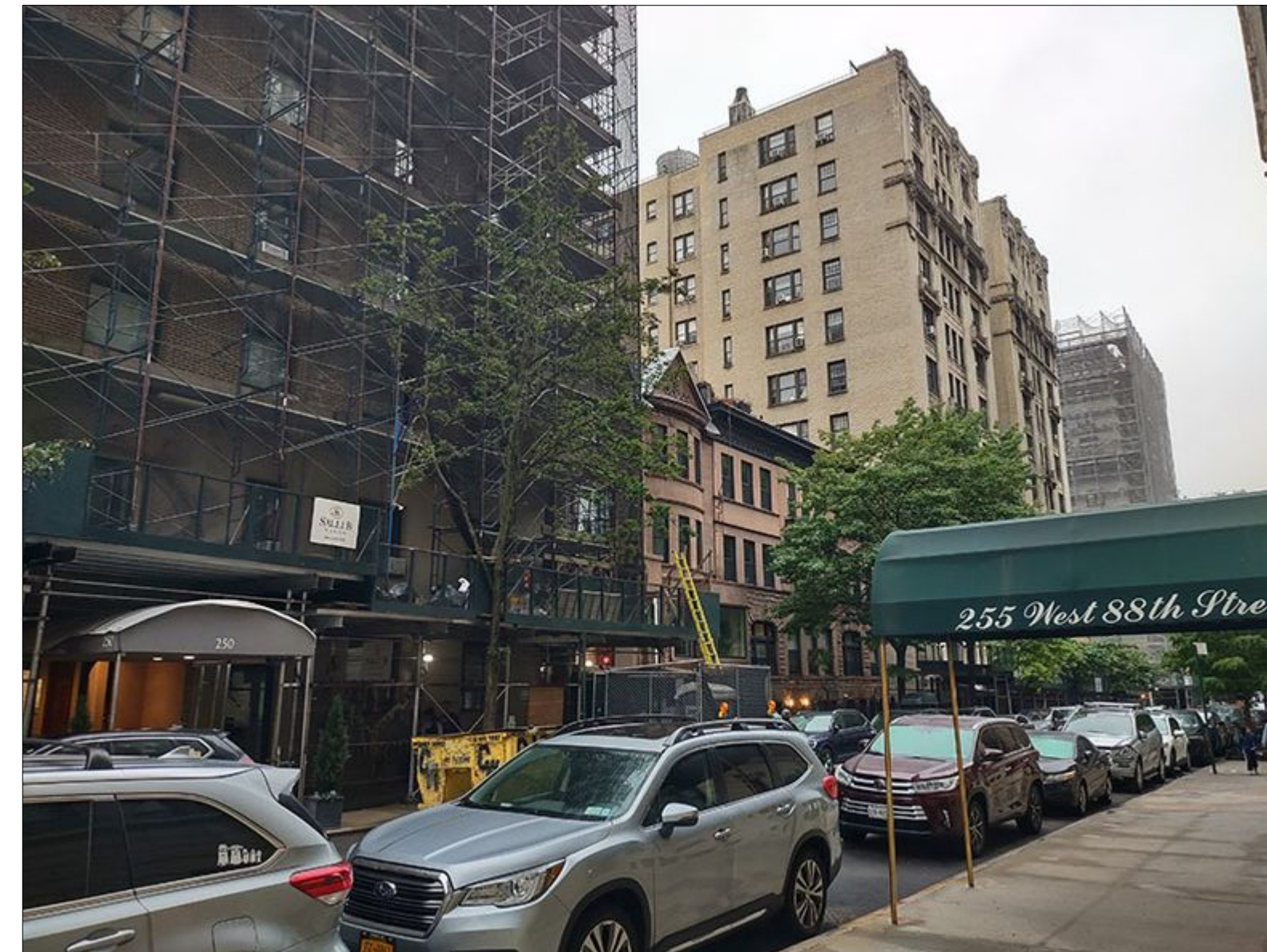
LOOKING SOUTH WEST 2
