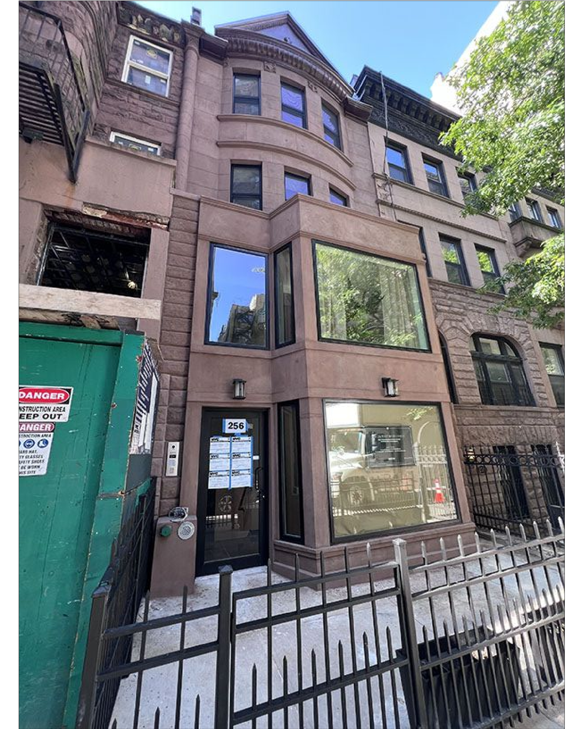
STOREFRONT- LOOKING SOUTH WEST
