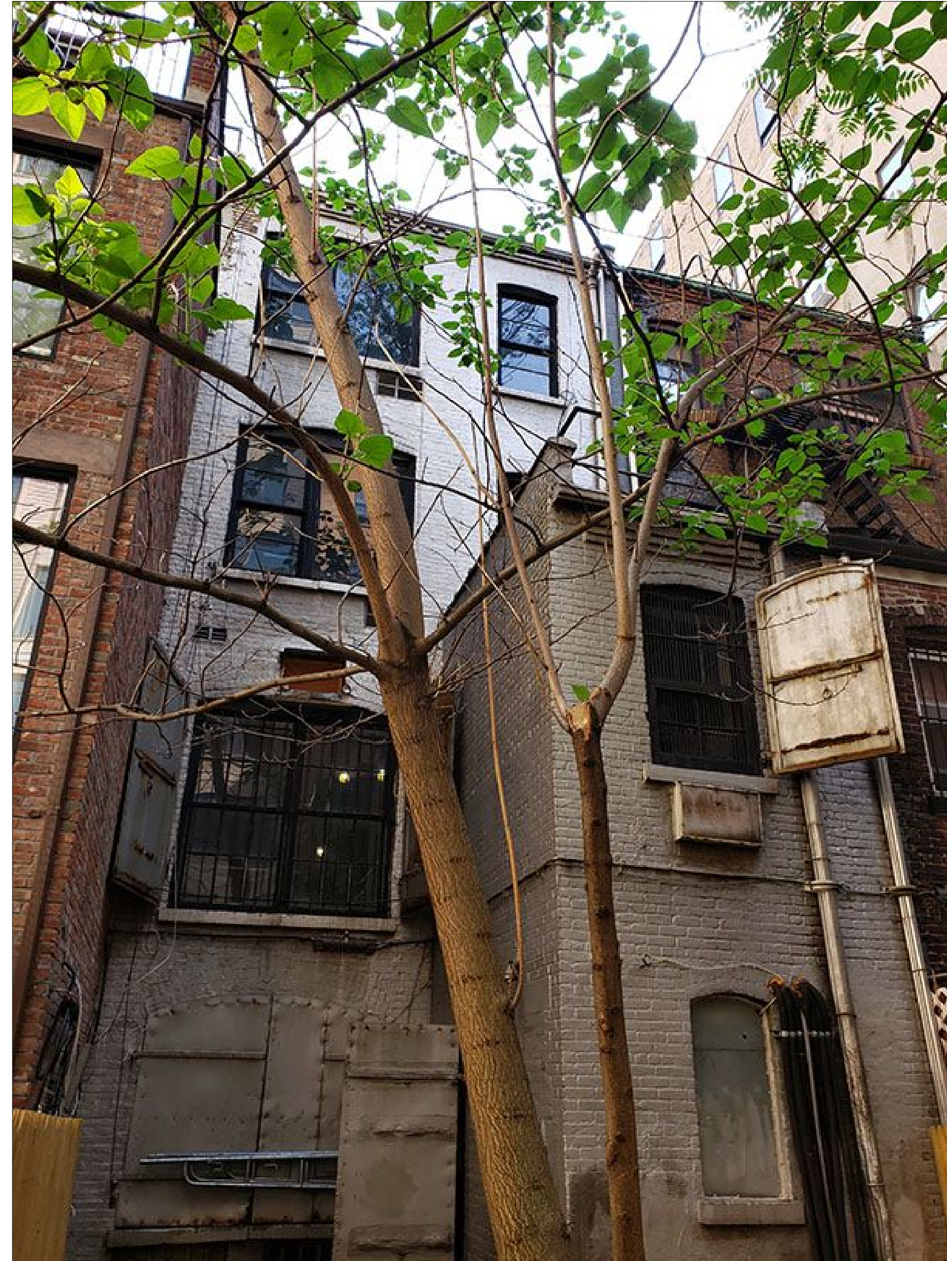
UPPER SOUTH FACADE PRIOR TO CONSTRUCTION
