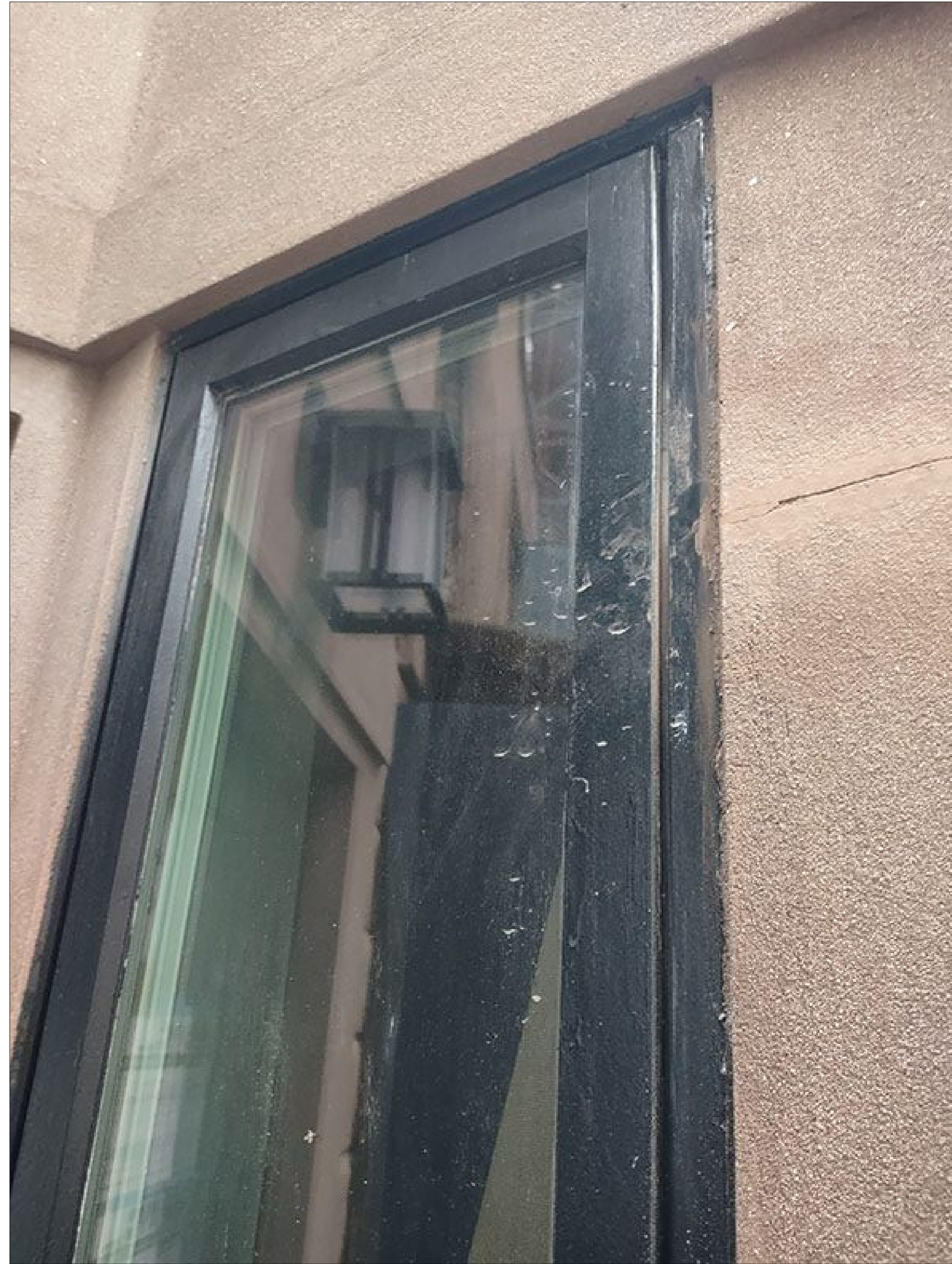
N.W. BASEMENT BAY WINDOW
