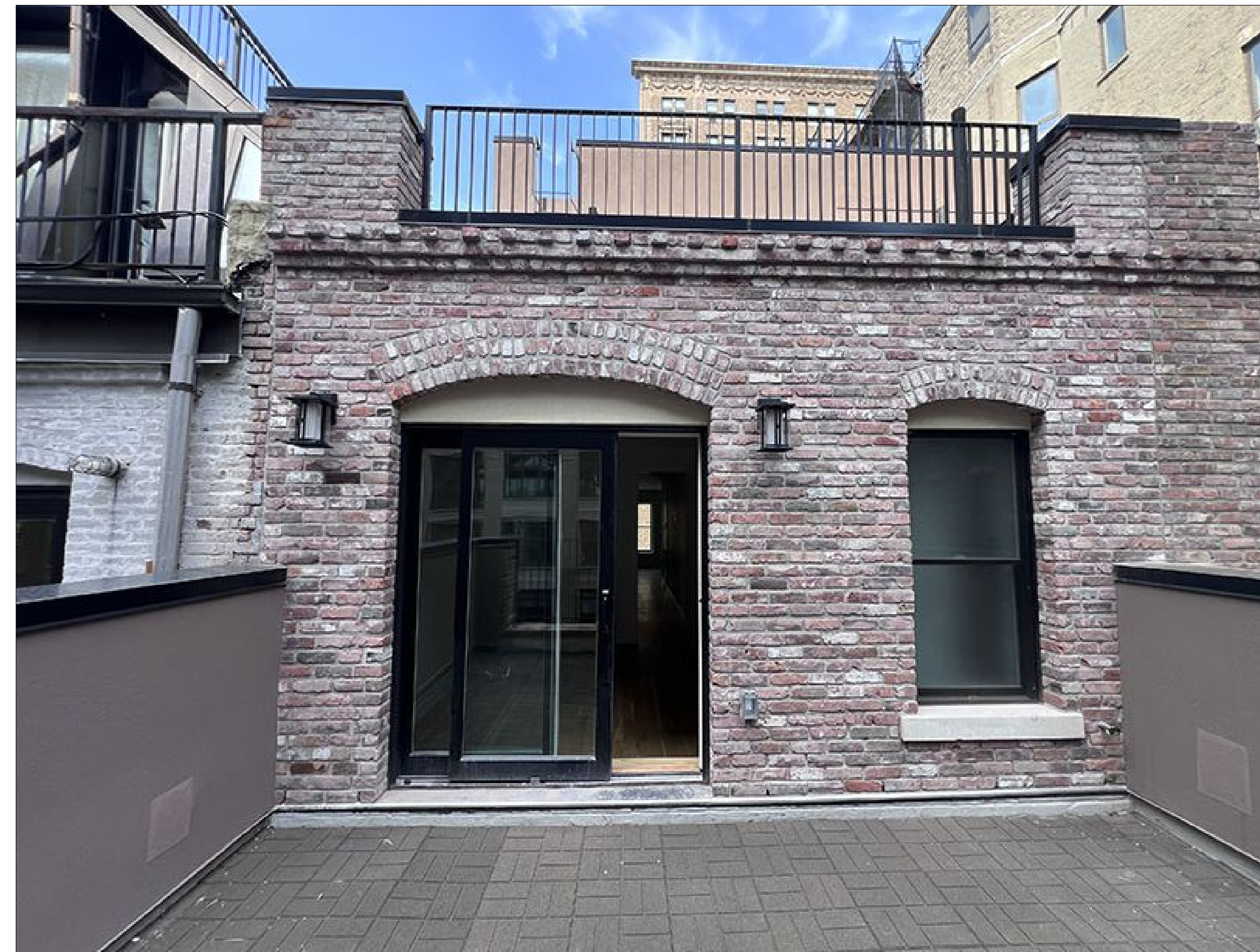
SOUTH FACADE @ 3RD FLOOR
