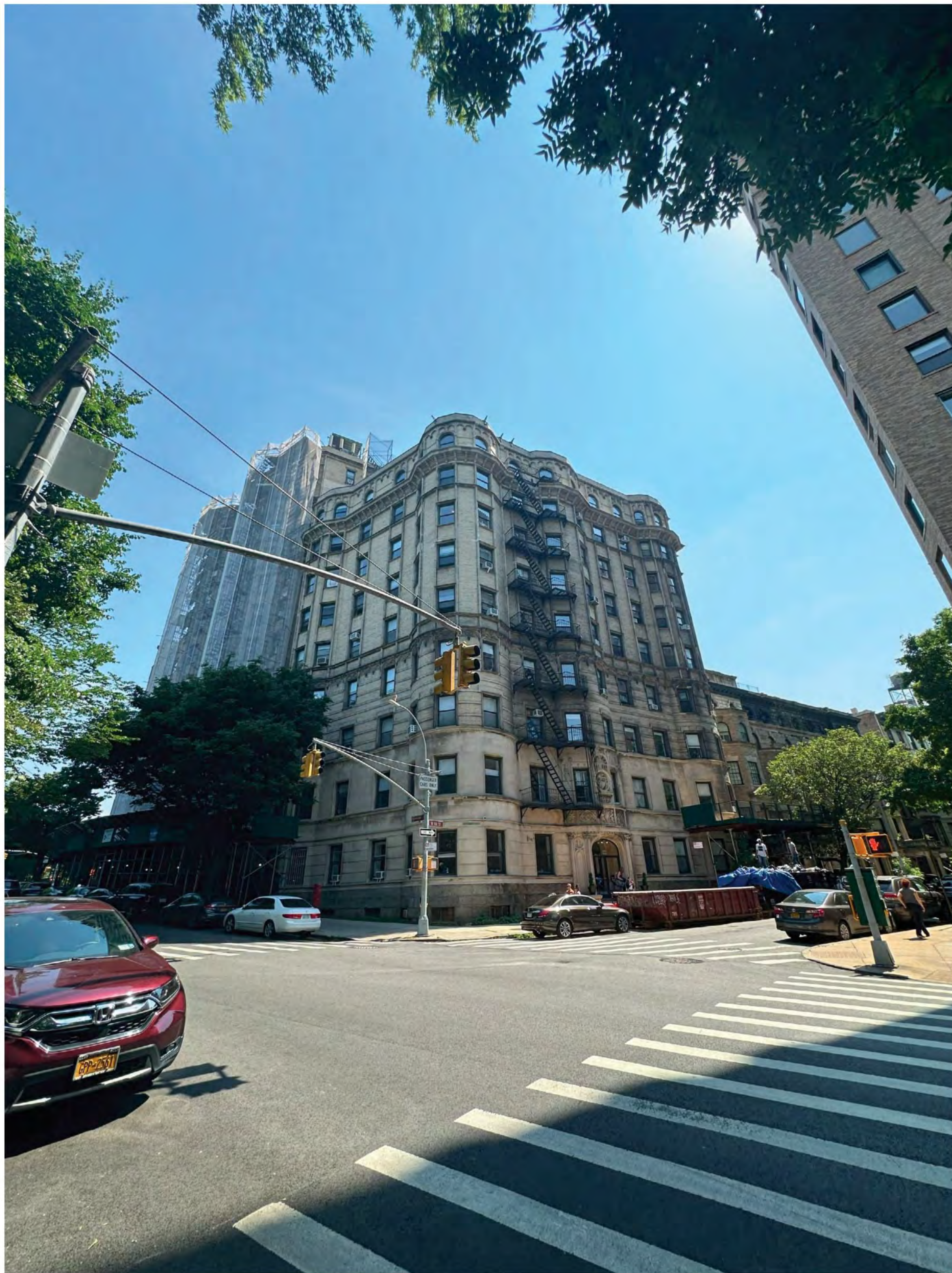
EXISTING WEST AND SOUTH SIDE VIEW
