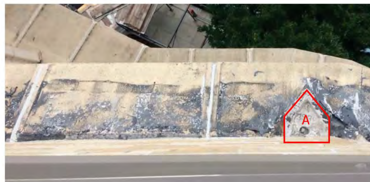
EXISTING PARAPET CONDITION
