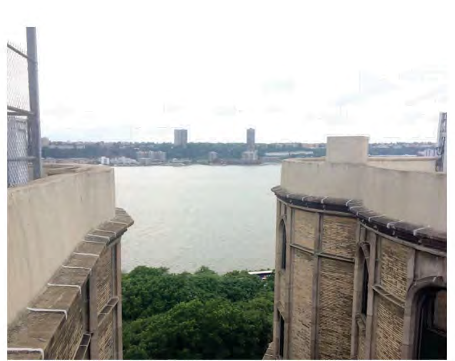
125 RIVERSIDE DRIVE PARAPET
