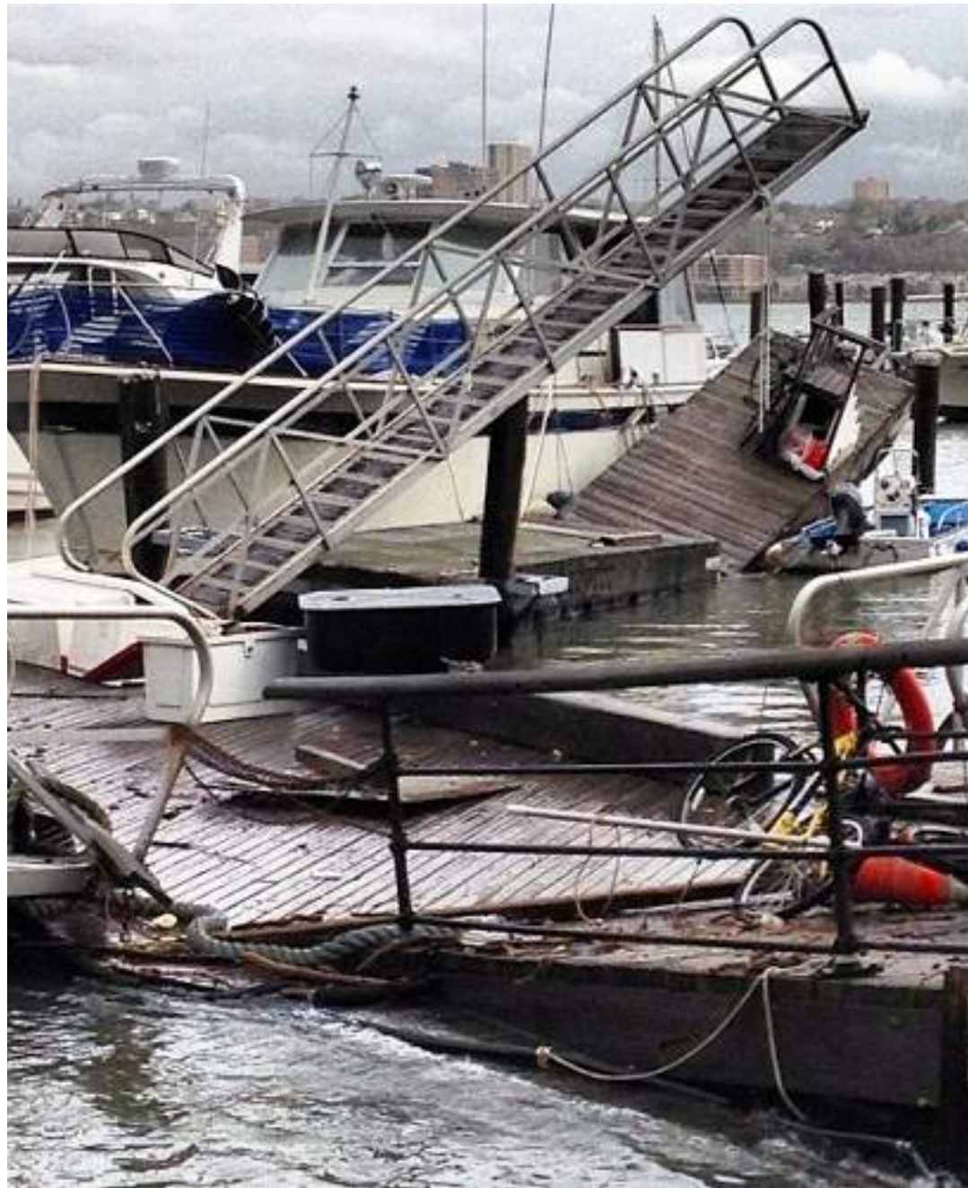
Dock & Gangway Damage
