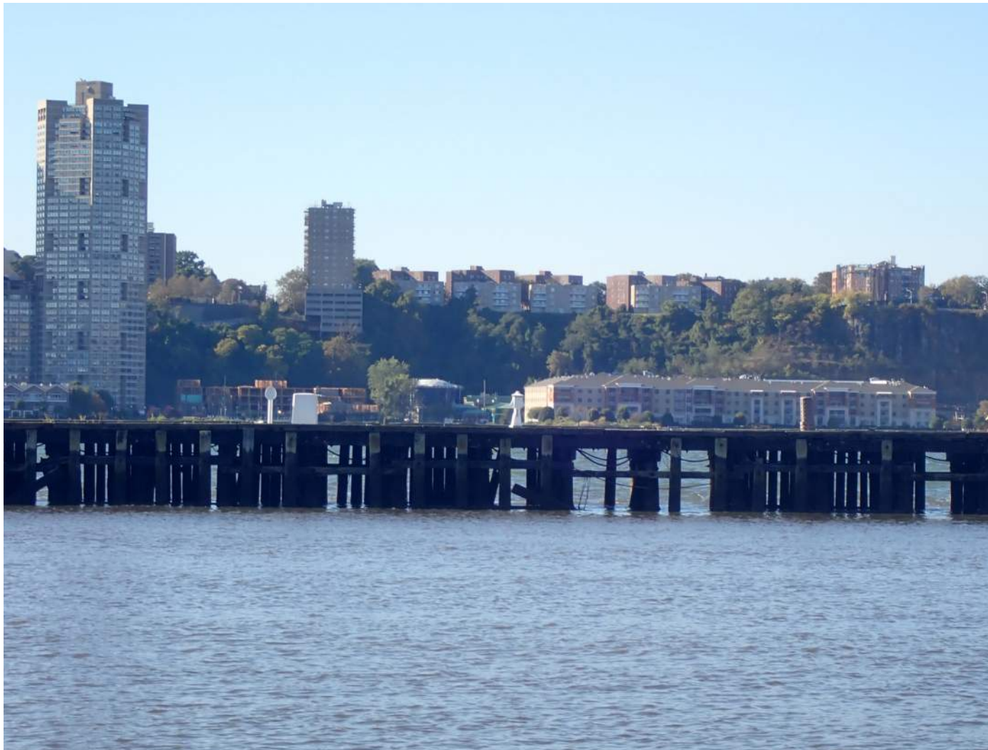
1 - View Looking West at Wave Screen
