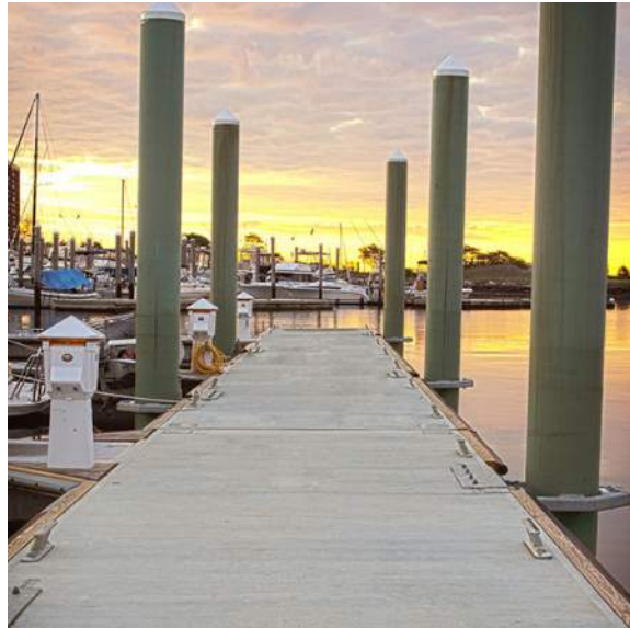
Floating Dock Pile Guides
