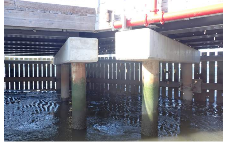
Steel Piles & Concrete Pile Caps
