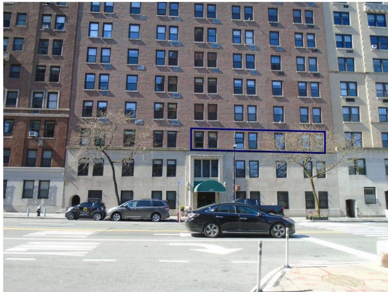
322 W 72nd Street - North Facade
