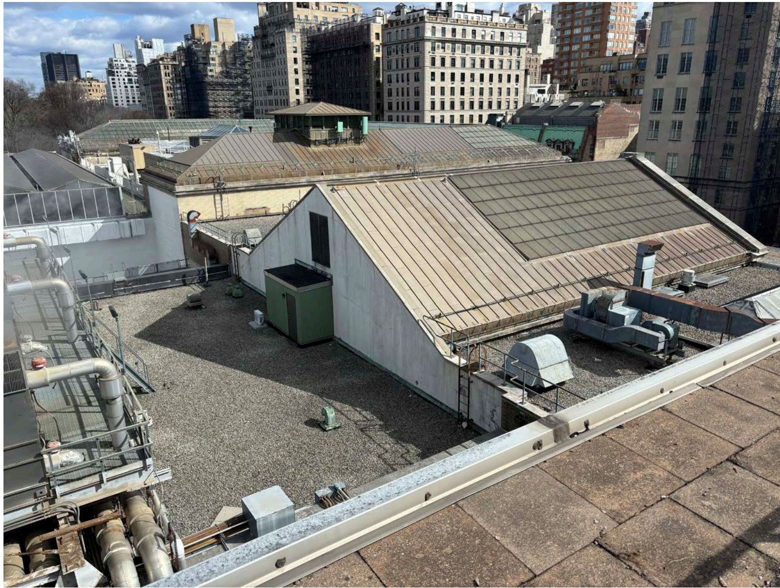
EXISTING CONDITION GRRR ROOF AND WING E ROOF
