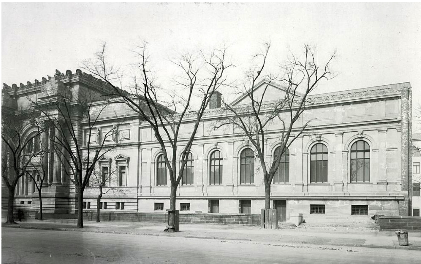
PHOTO OF WING E AROUND 1912. THE BOILER HOUSE CHIMNEY IS VISIBLE LEFT OF THE PEDIMENT.
