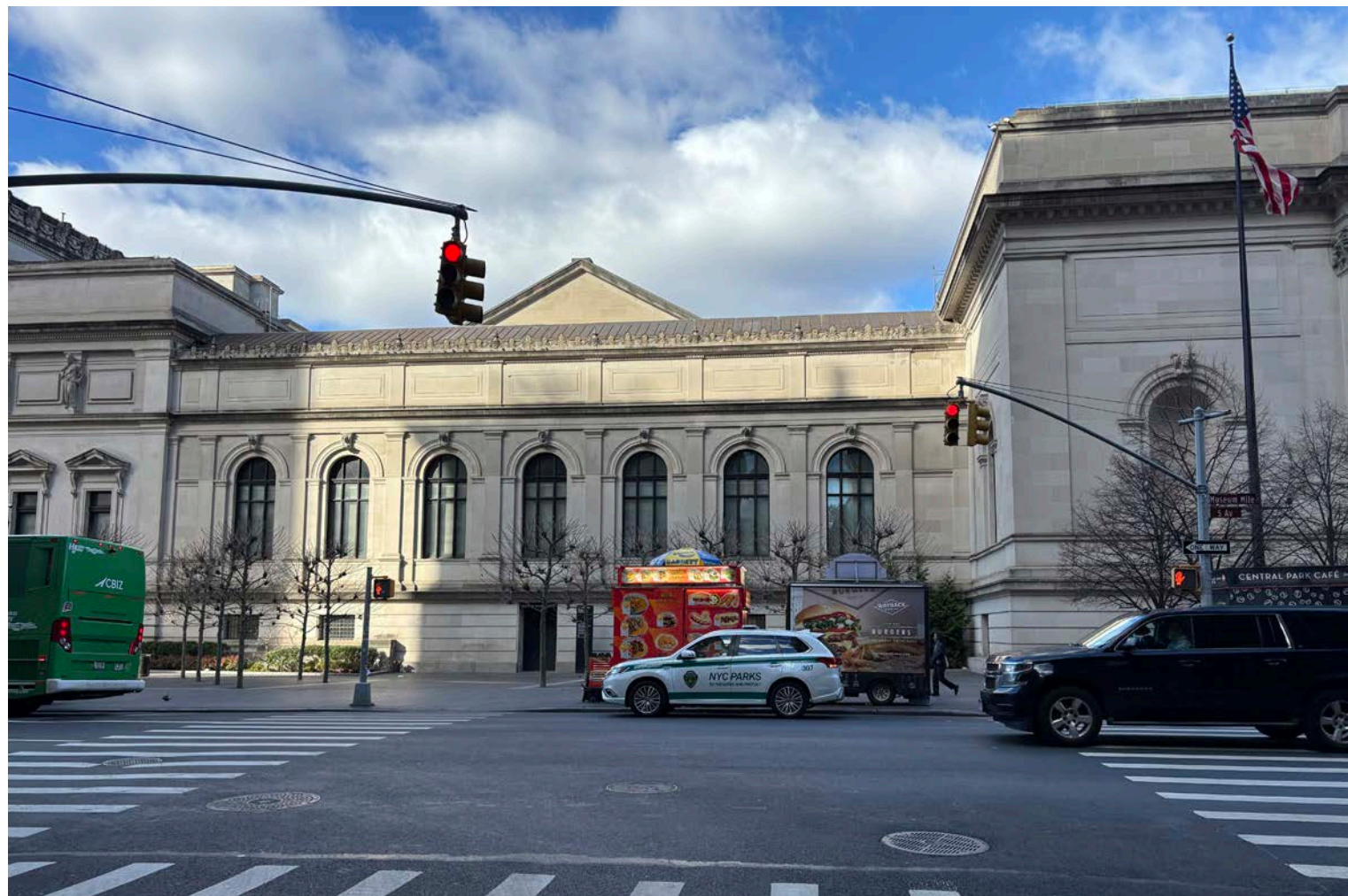
THE SCREEN WALL AT THE NORTH SIDE COOLING TOWERS WILL NOT BE VISIBLE ABOVE WING E ROOF WHEN CLOSE TO THE BUILDING AT THE PLAZA OR FIFTH AVENUE.
