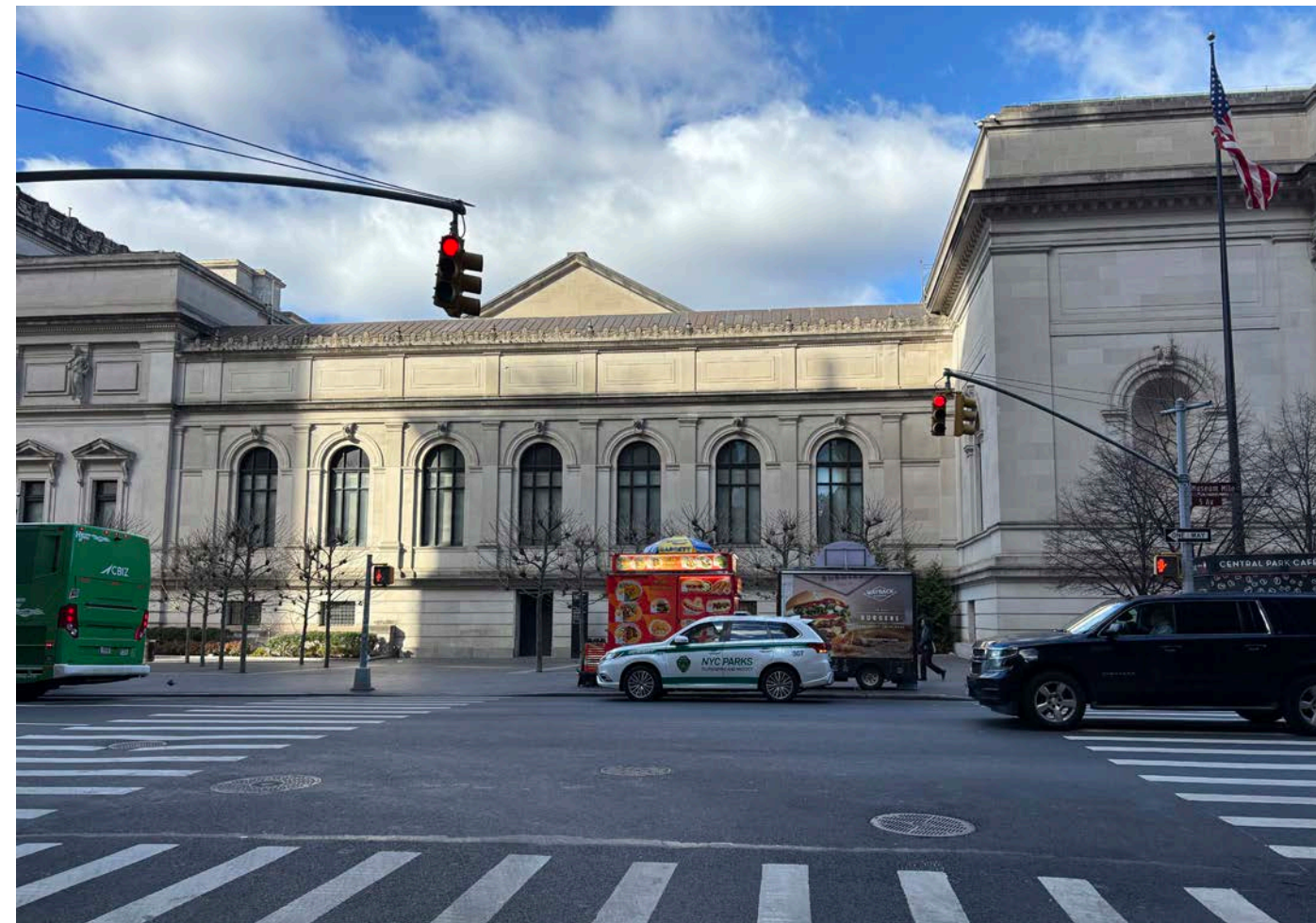
EXISTING CONDITION PHOTO VIEW 1
