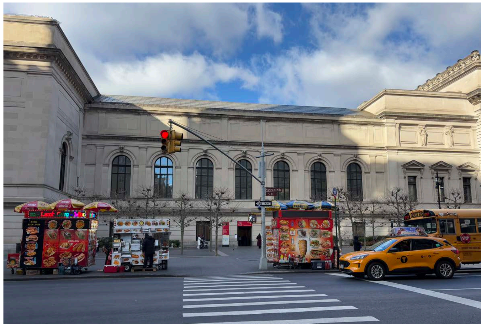
THE EXISTING SCREEN WALL AT THE SOUTH SIDE COOLING TOWERS IS NOT VISIBLE WHEN CLOSE TO THE BUILDING AT THE PLAZA OR FIFTH AVENUE.
