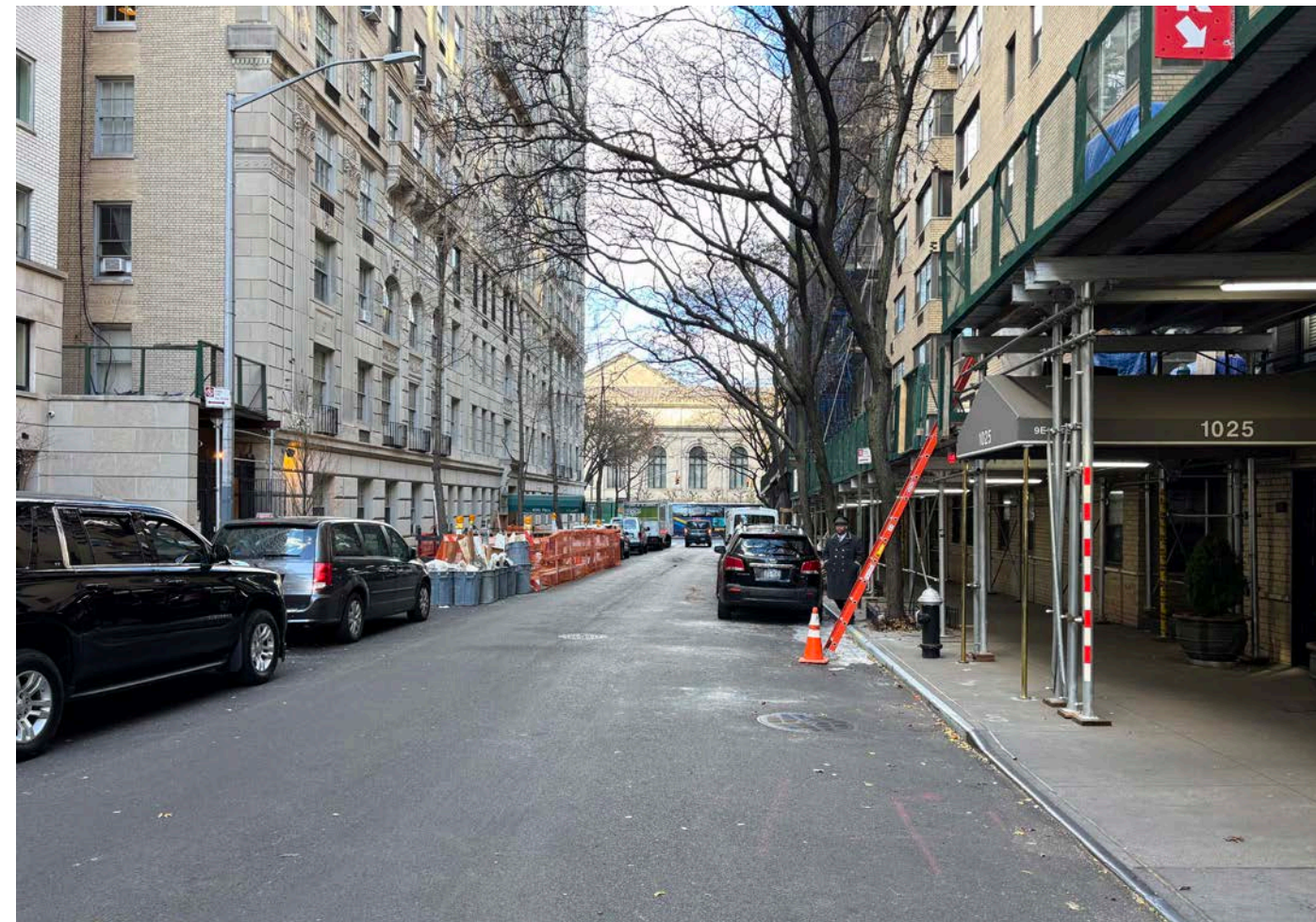
EXISTING CONDITION PHOTO VIEW 4
