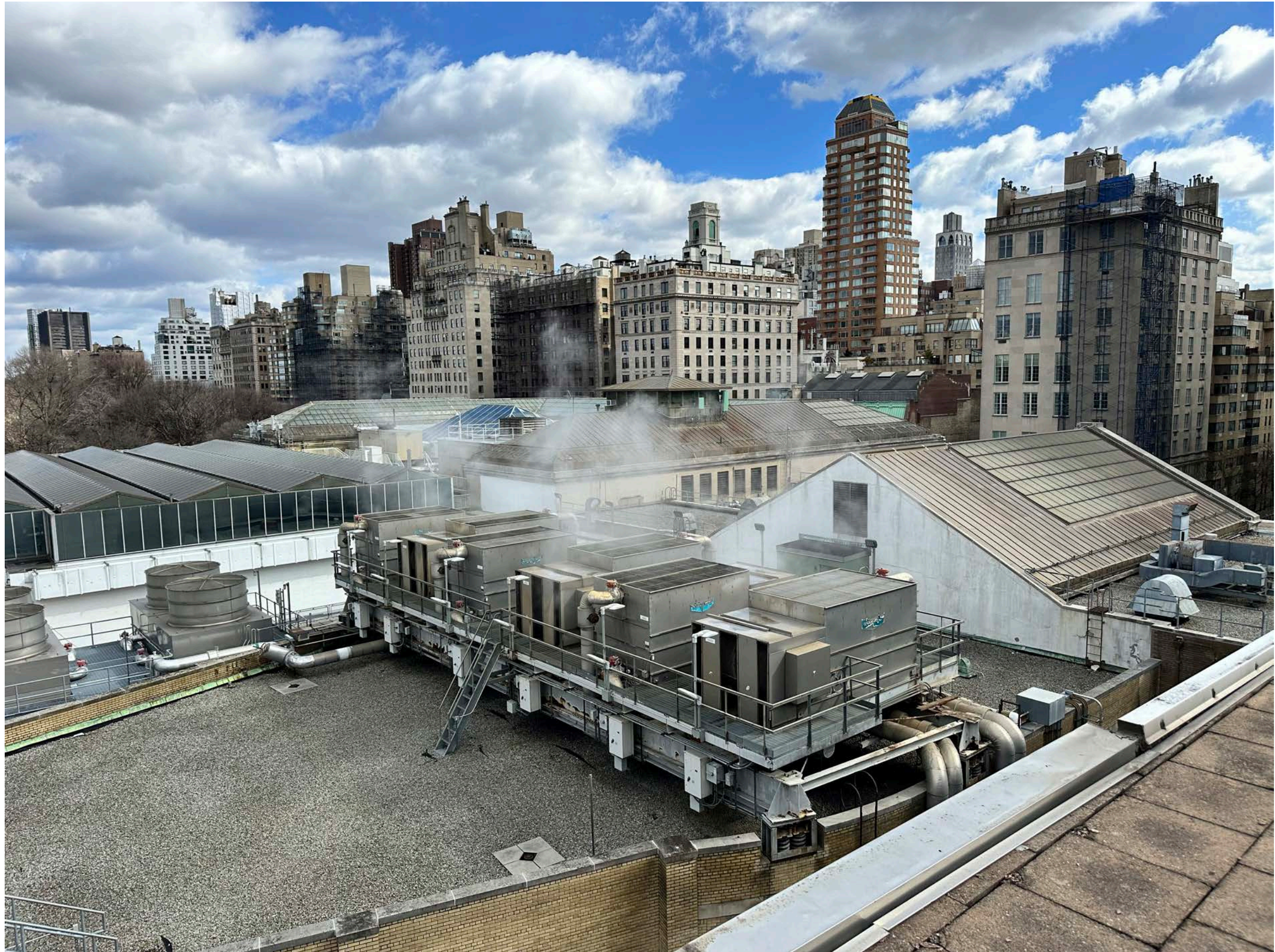
EXISTING CONDITION GRACE RAINEY ROGERS AUDITORIUM ROOF AND COOLING TOWERS
