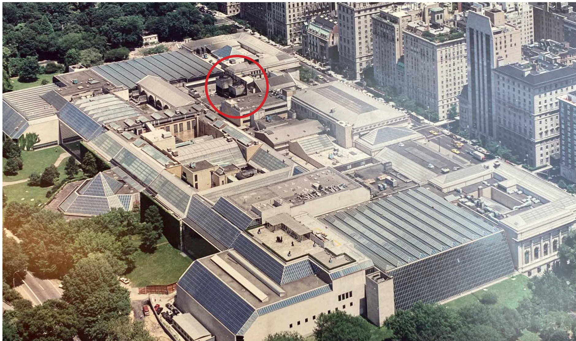
AERIAL VIEW 1991, SHOWING COOLING TOWERS AND SCREEN WALL ON ROOF OF GRACE RAINEY ROGERS AUDITORIUM
