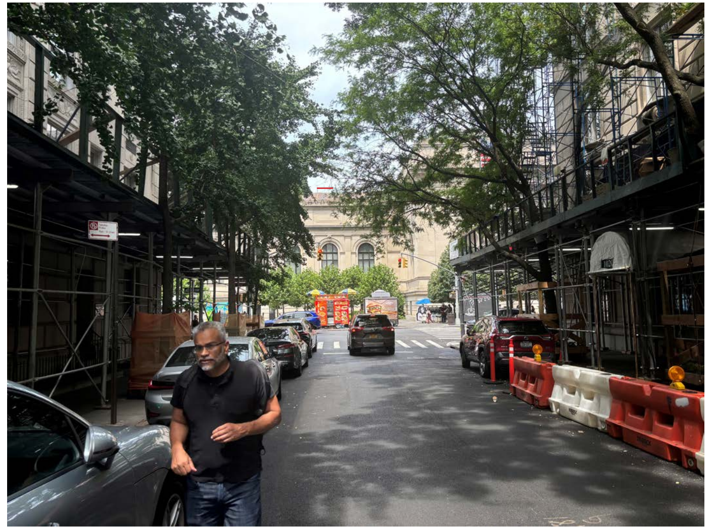
PHOTO ON E 83RD ST SOME DISTANCE FURTHER DOWN THE STREET
