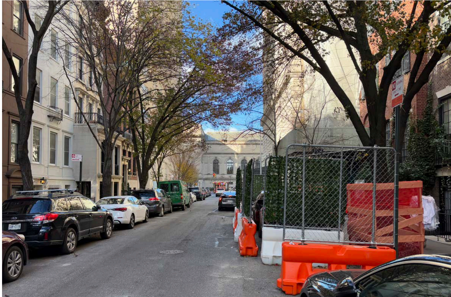
THE EXISTING SCREEN WALL AT THE SOUTH SIDE COOLING TOWERS IS PARTIALLY VISIBLE ABOVE THE WING J ROOF VIEWED FROM FARTHER DOWN THE SIDE STREET (E. 81ST ST).
