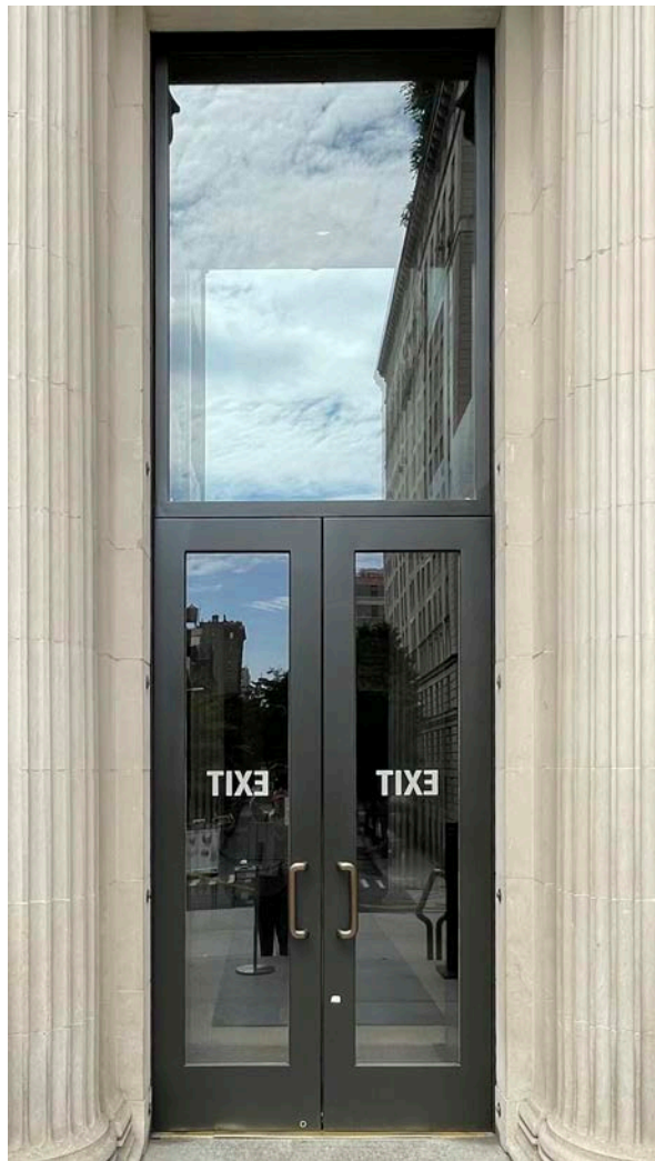
PHOTO SHOWING EXISTING 82ND DOORS
