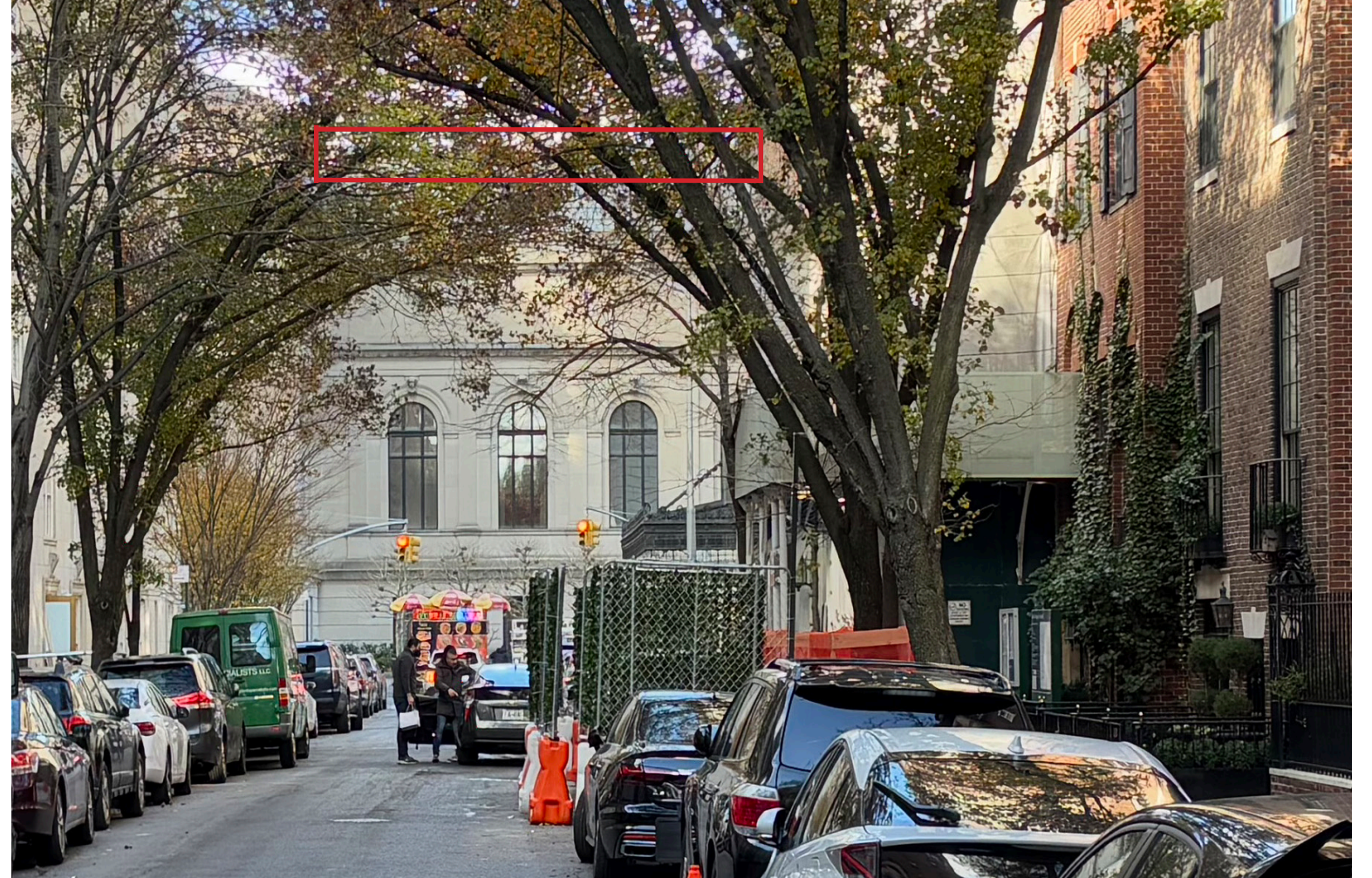
ENLARGED DETAIL OF PHOTO AT LEFT SHOWING EXISTING SCREEN WALL VISIBILITY ABOVE ROOF OF WING J (HIGHLIGHTED WITH RED LINE)
