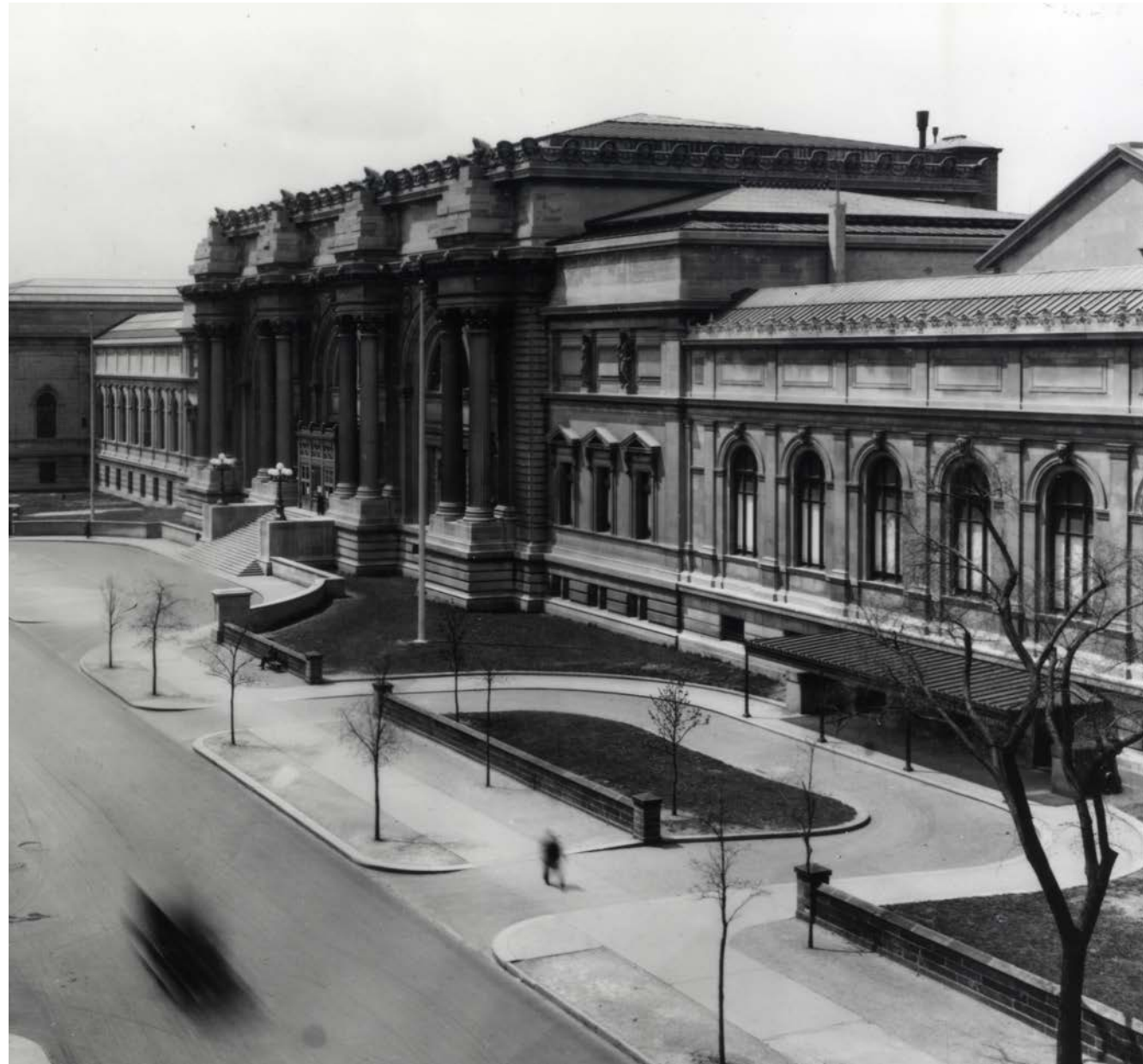
PHOTO 1 - LOOKING SOUTH WEST SHOWING ORIGINAL MARQUEE AT WING E - 83RD ST ENTRANCE
