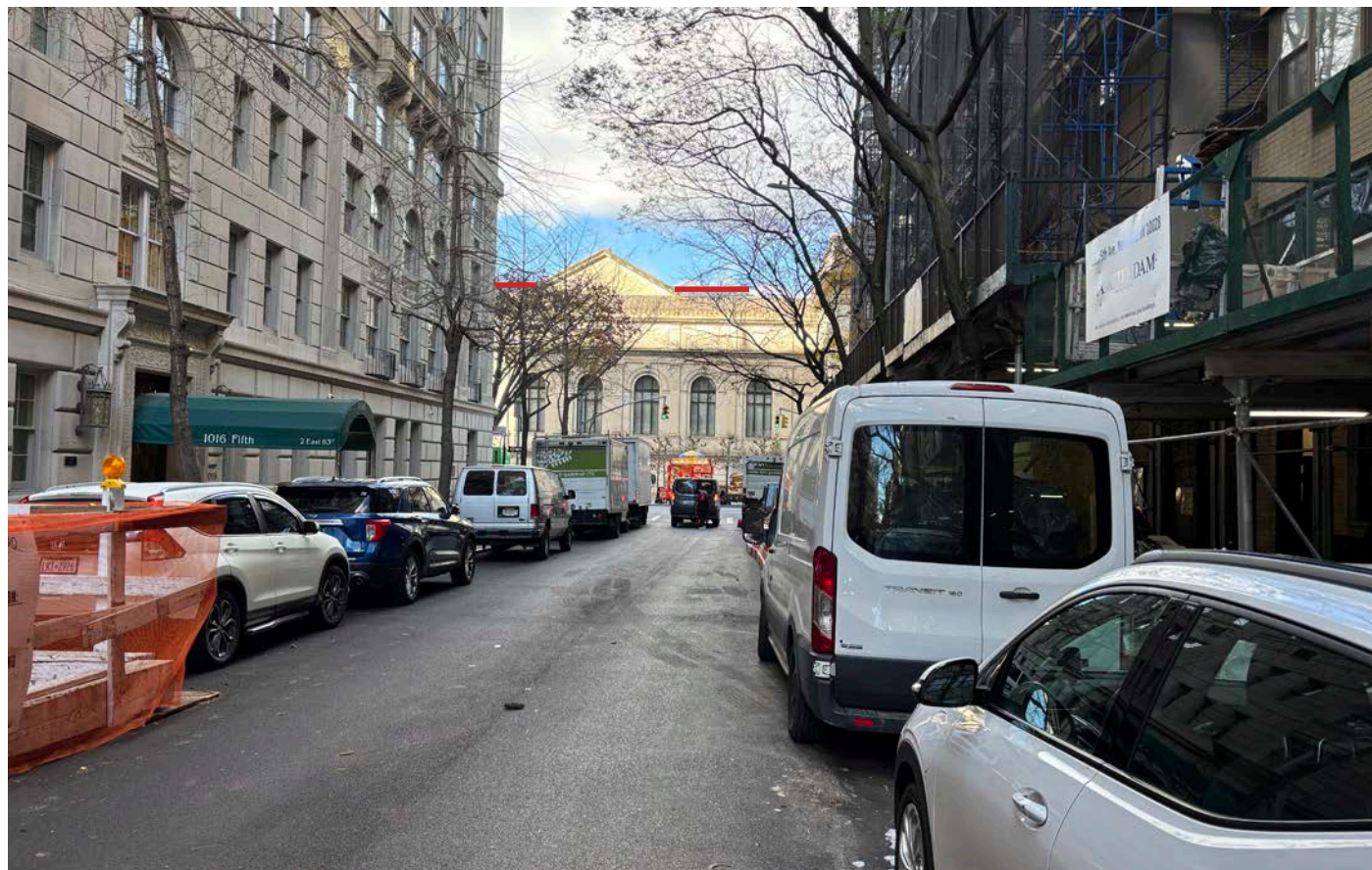
MONTAGE VIEW 3 - TOP OF SCREEN WALL VISIBLE HIGHLIGHTED WITH RED LINE RESTORATION OF THE 83RD STREET ENTRANCE AND NORTHSIDE CHILLER PLANT REPLACEMENT
