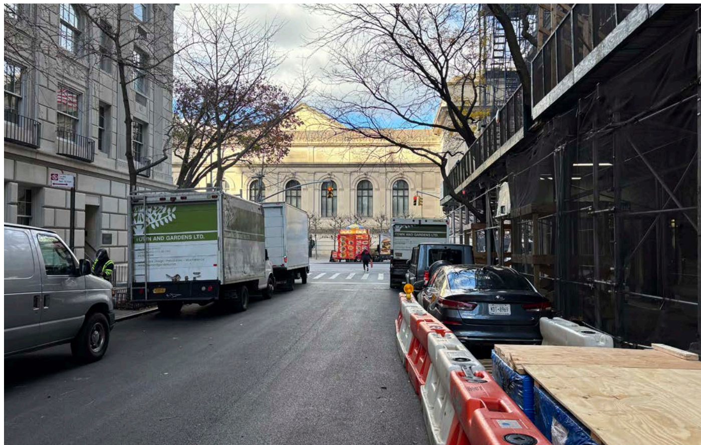
MONTAGE VIEW 2 - TOP EDGE OF SCREEN WALL BECOMES VISIBLE (RIGHT OF PEDIMENT)
