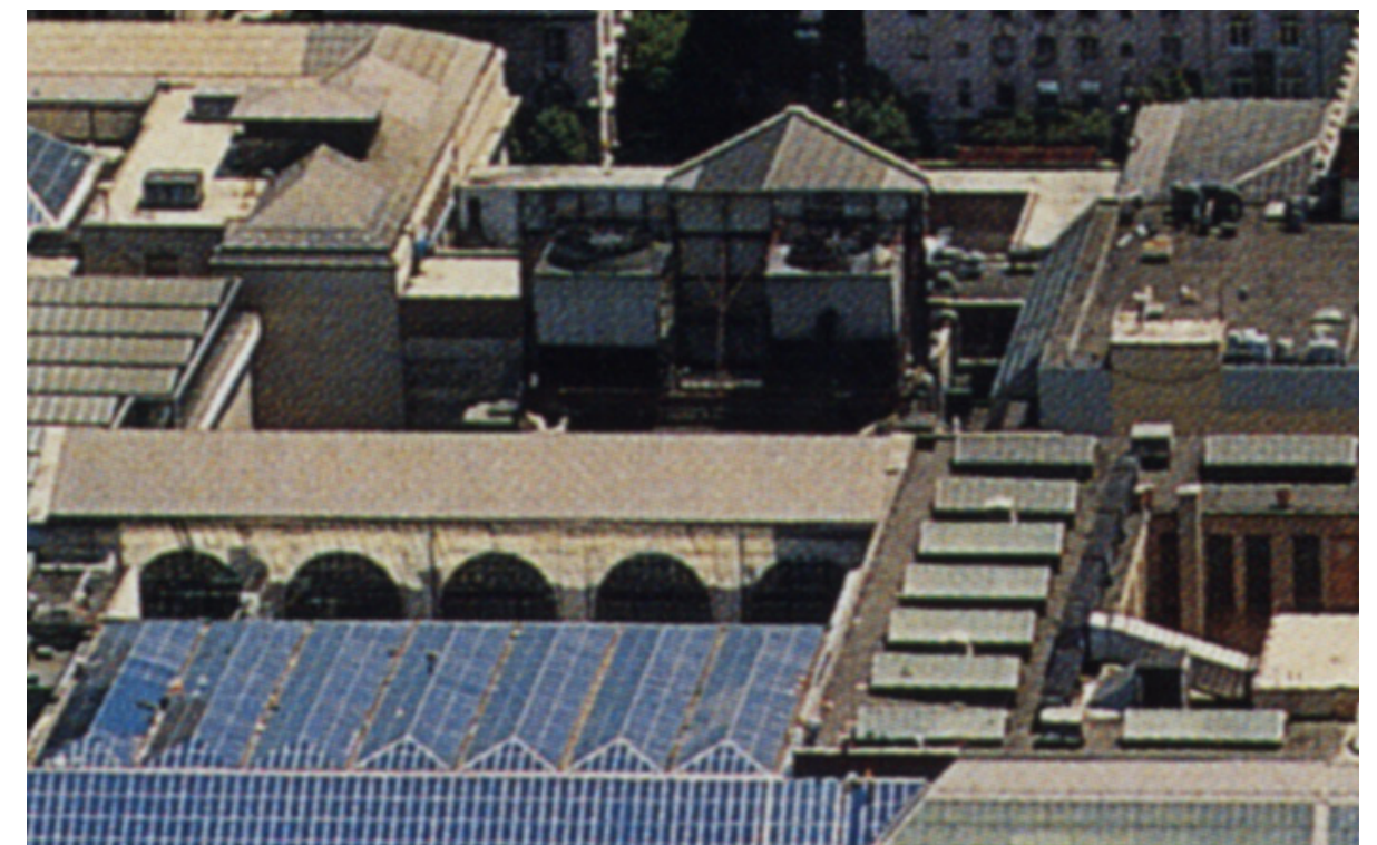
DETAIL SHOWING COOLING TOWERS AND SCREEN WALL ON ROOF
