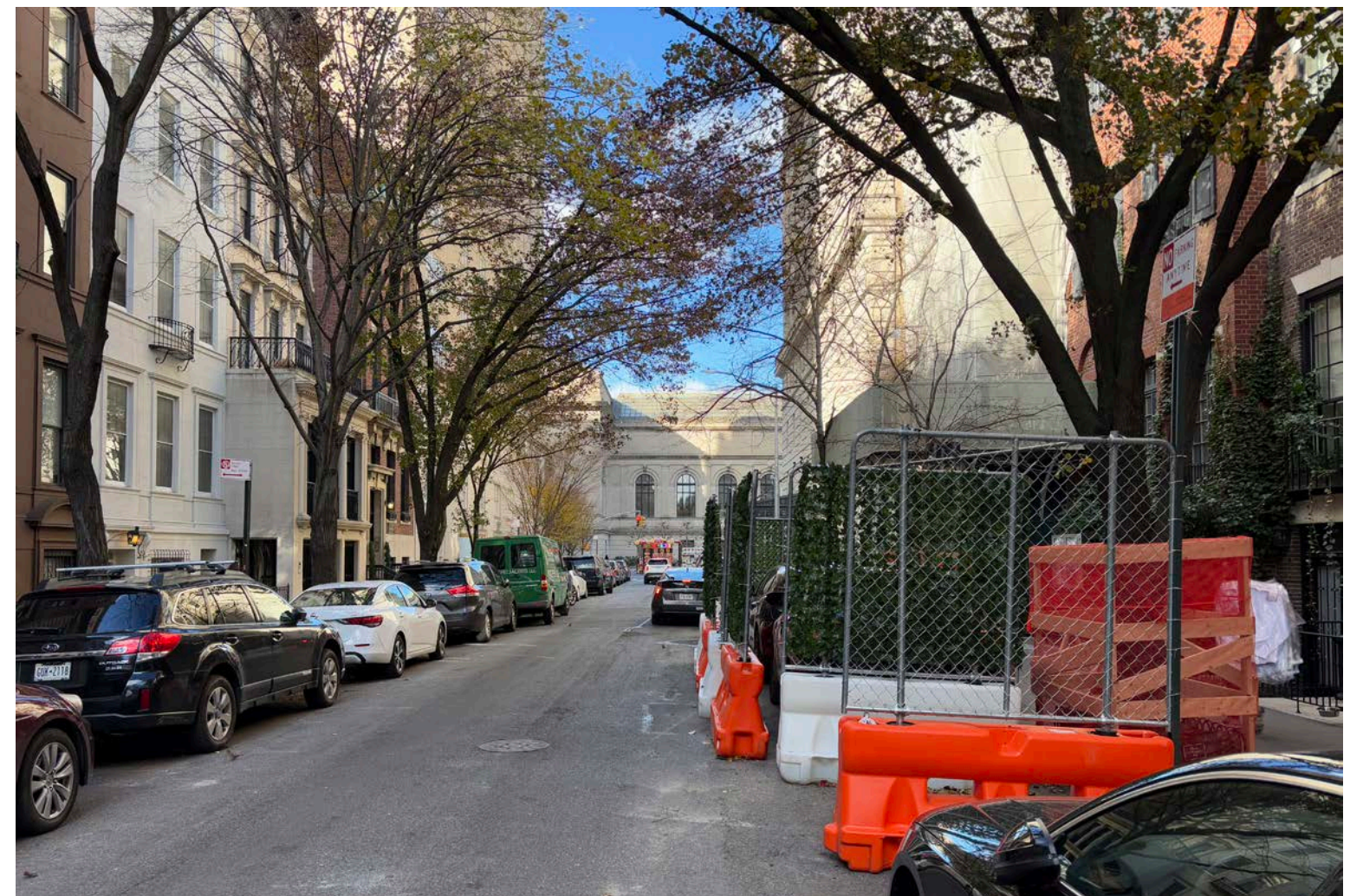
THE EXISTING SCREEN WALL AT THE SOUTH SIDE COOLING TOWERS IS PARTIALLY VISIBLE ABOVE THE WING J ROOF VIEWED FROM FARTHER DOWN THE SIDE STREET (E. 81ST ST).
