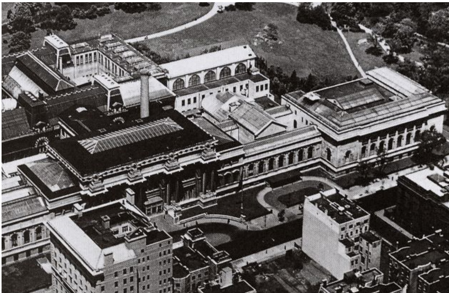
AERIAL VIEW 1920'S. BOILER HOUSE CHIMNEY IS VISIBLE.
