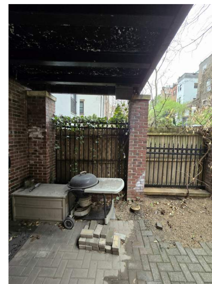
garden level under deck looking east.
