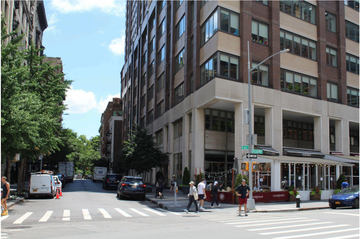
Figure 1. View towards proposed Link 5G tower, on the corner of Broadway and West 64th Street, taken from the Broadway Mall, 64th Street. The West Side Y.M.C.A and the Society for Ethical Culture viewed towards the end of the south side of West 64th Street and the southwest corner of Central Park West and West 64th Street.
