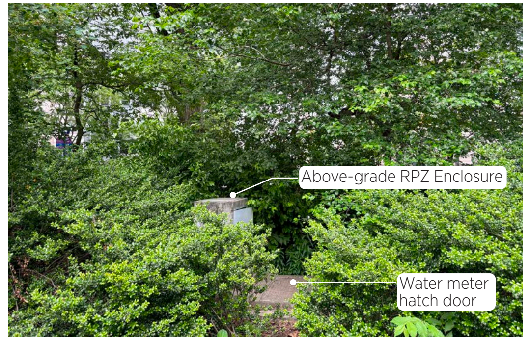
RPZ AND WATER METER (TYPICAL CONDITION)
