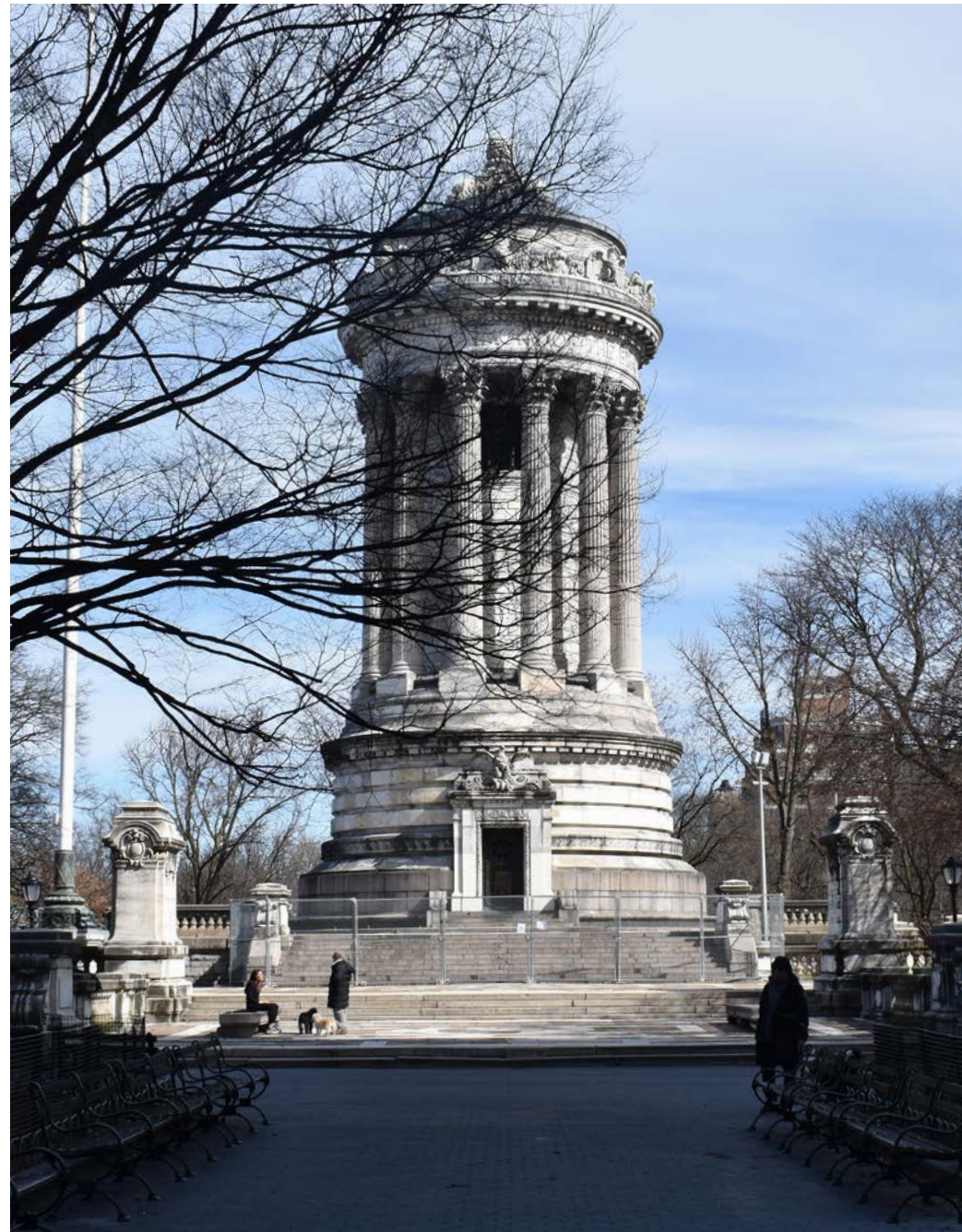
2— View from South Plaza, 2024
