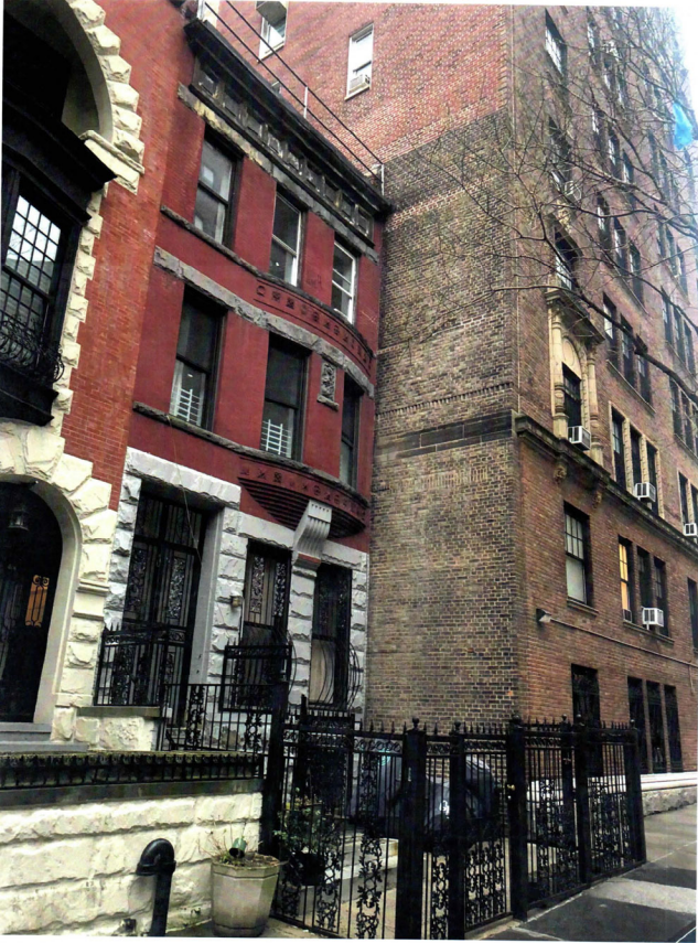
CONDITIONS BEFORE WORK
