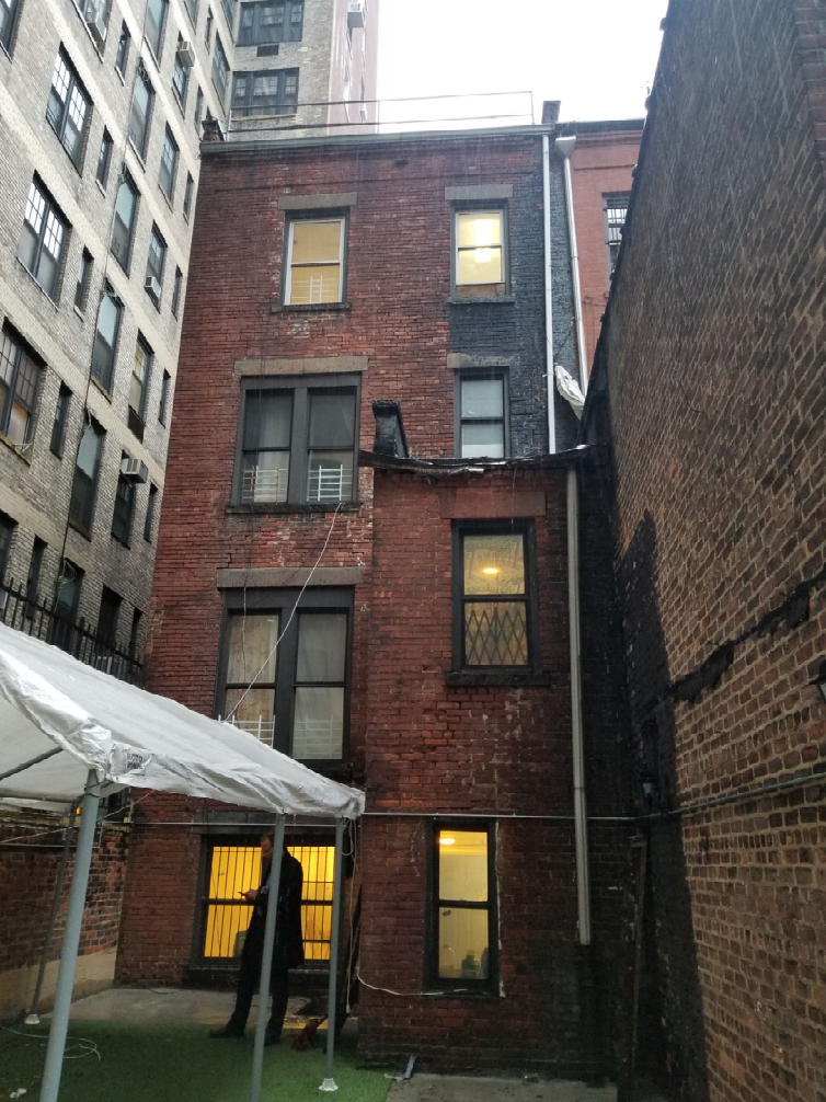
CONDITIONS BEFORE WORK
