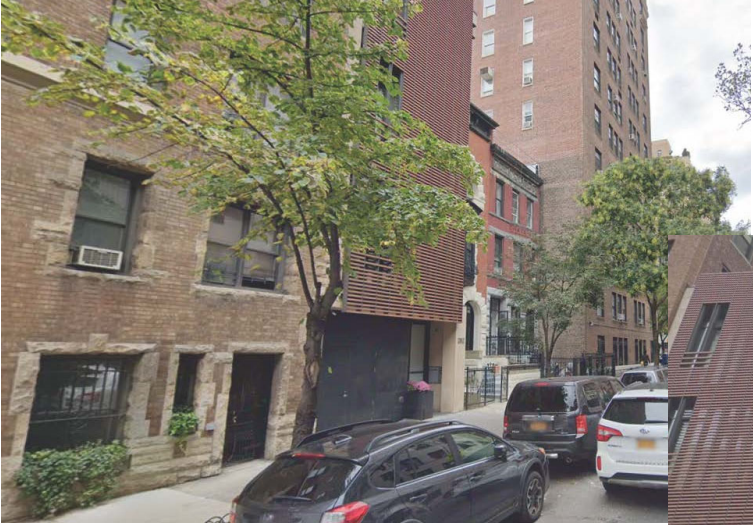
VIEW FROM EAST CORNER OF 75 STREET
