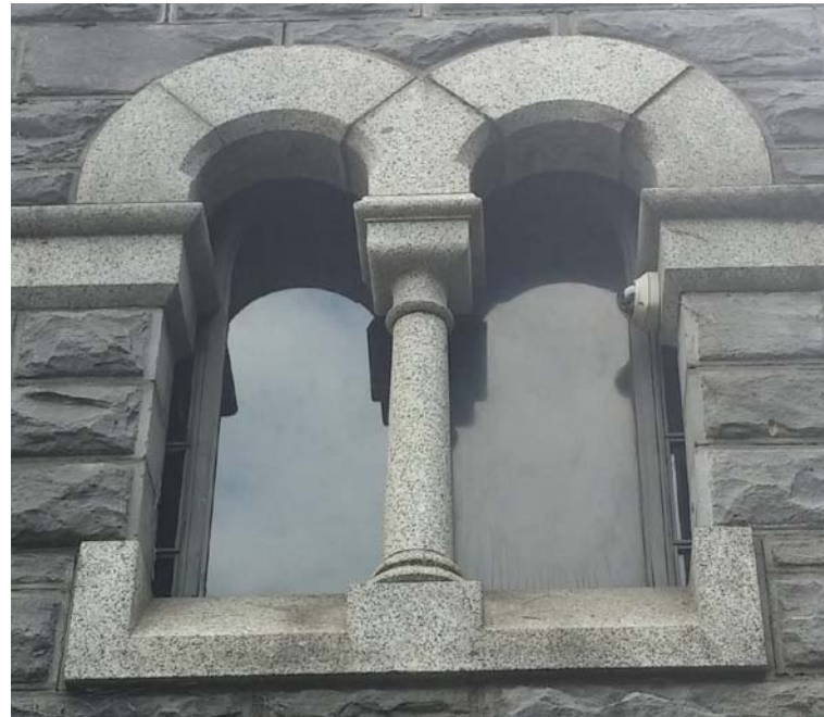
W2 EXISTING EXTERIOR
