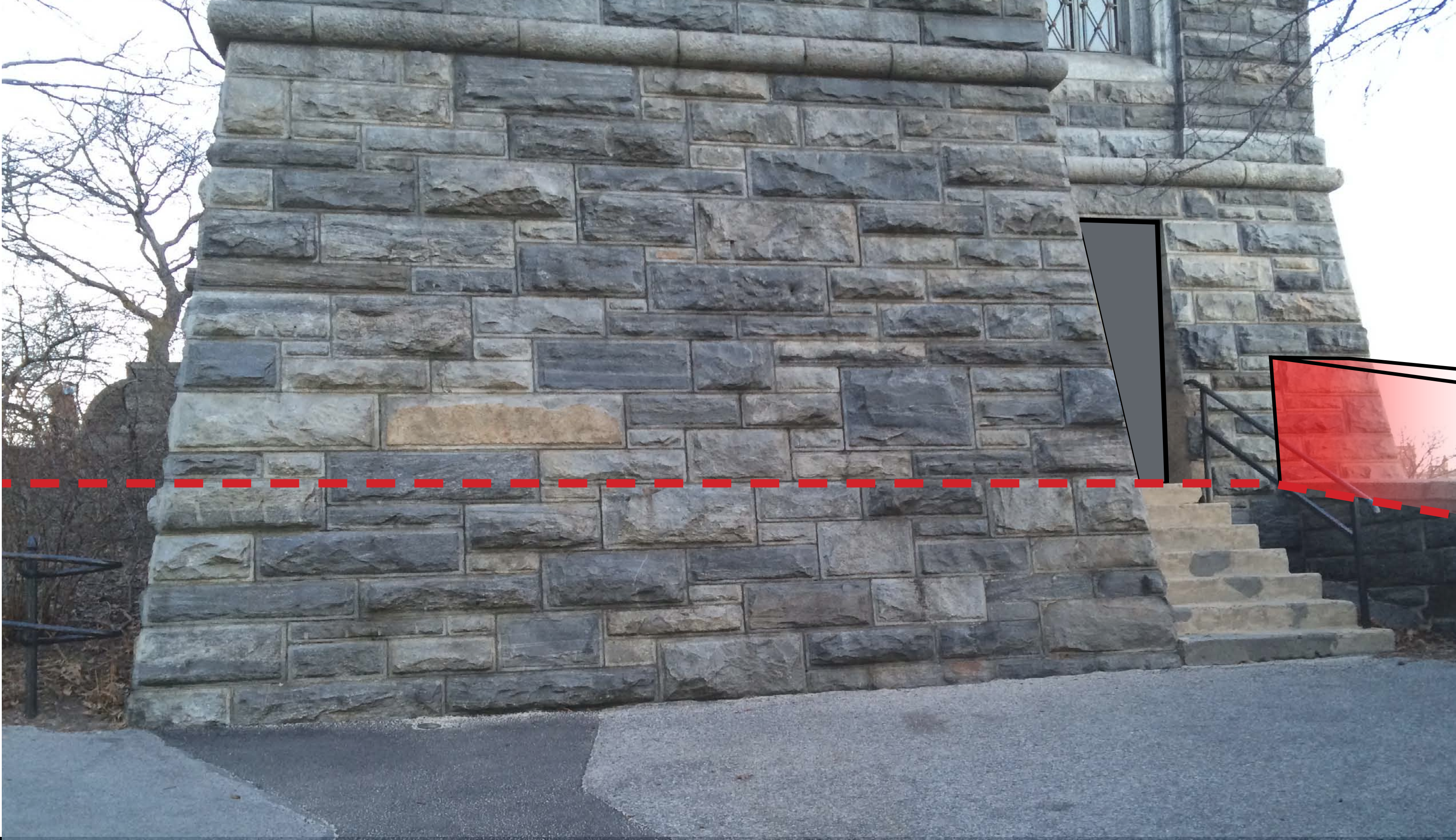
Proposed Grade Change at Basement Entrance
