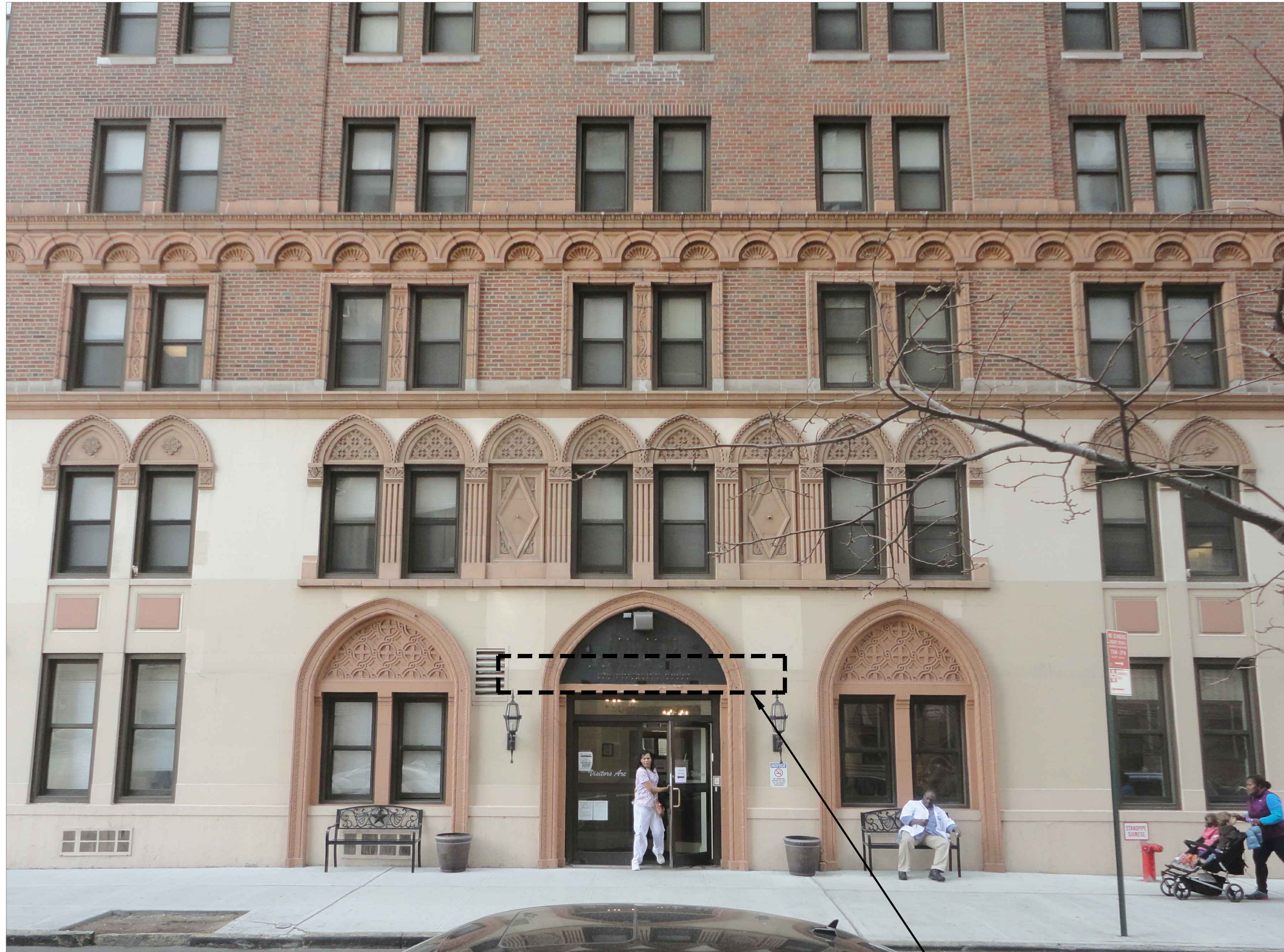
2 EXISTING CONDITION - ENTRY (W. 87TH STREET) N.T.S.
